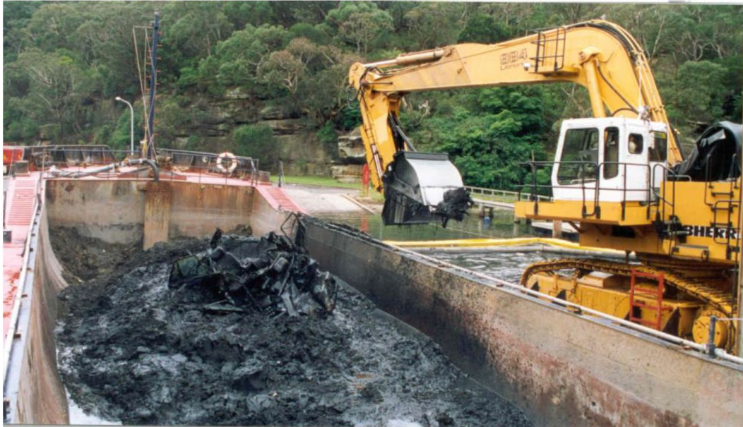
Figure 7-1: Example backhoe dredge loading hopper barge with closed 'bucket' (environmental clamshell) attachment
