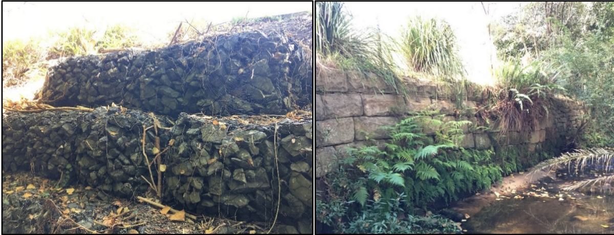
Figure 3-16 Burnt Bridge Creek rock gabion (left) and rock wall (right)
