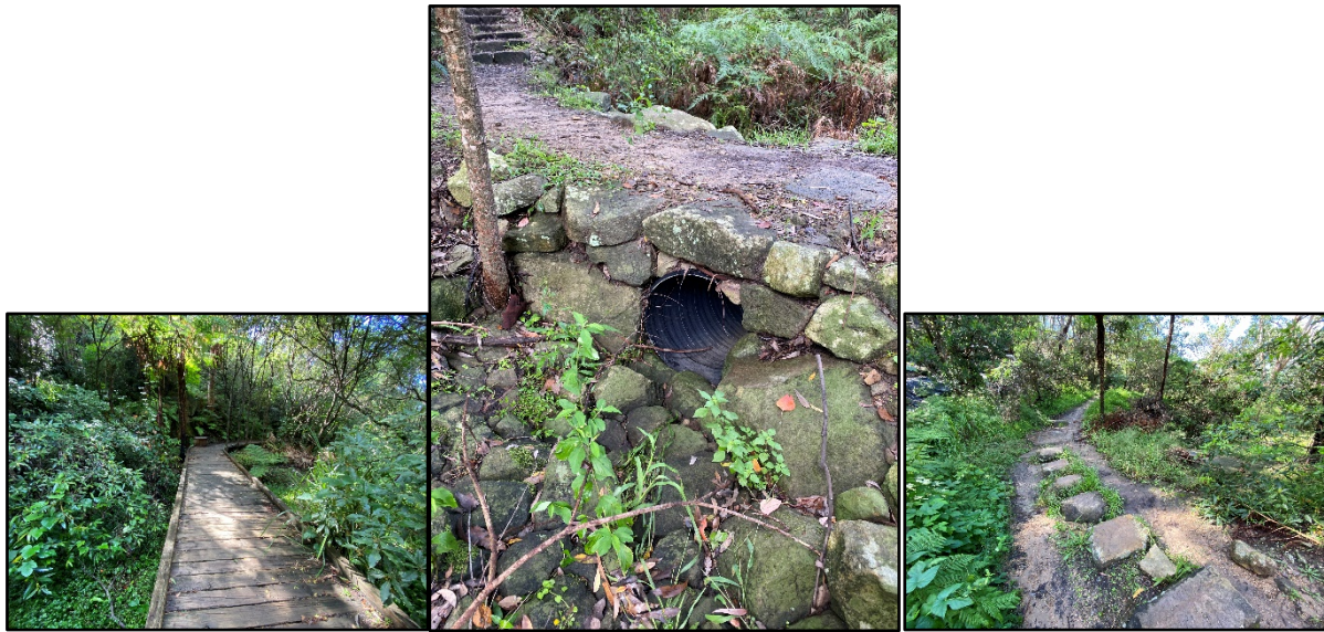
Figure 3-6 Wilksch Walk crossings along the existing aboveground watercourse
