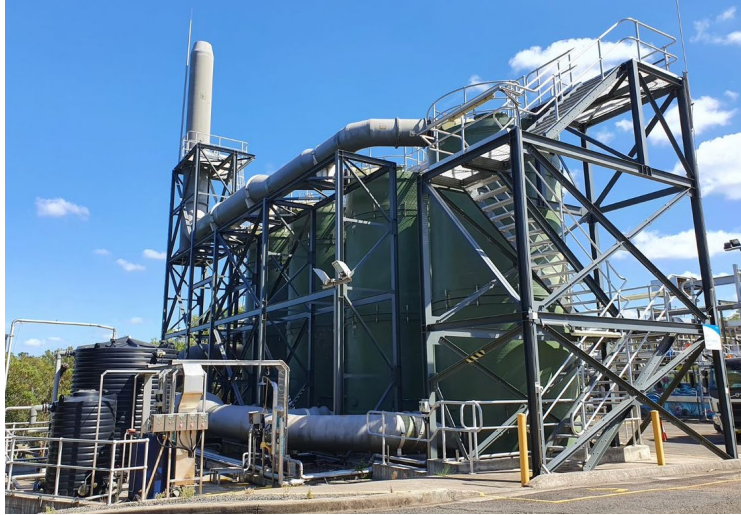
Figure 4-4 Example odour control unit from an existing Sydney Water facility
