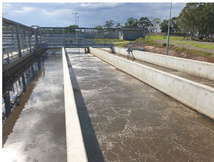
Figure 4-5 Example primary treatment area from an existing Sydney Water facility
