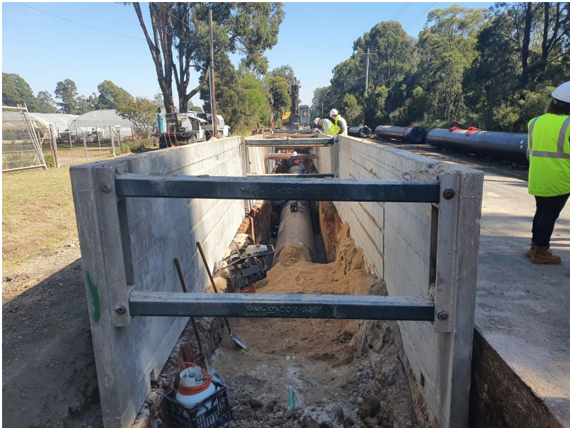
Figure 4-18 Trenched pipeline construction with shoring
