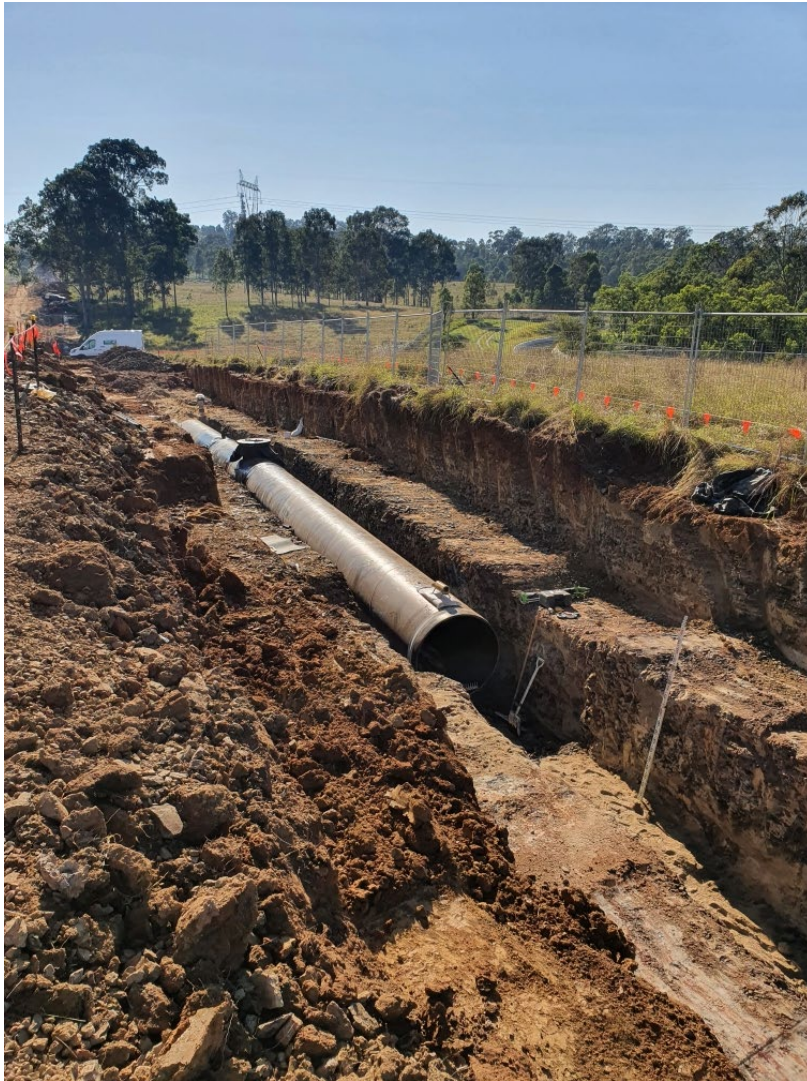
Figure 4-19 Trenched pipeline construction with benching
