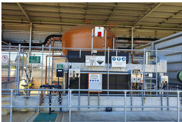
Figure 4-2 Example chemical storage area from an existing Sydney Water facility
