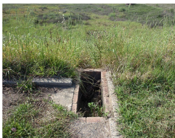
Figure 86. View south of brick lined sump forming part of an overflow channel on the reservoir wall, southern side of reservoir.
