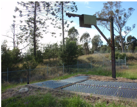
Figure 77. View south-east of a winch and grate system on the eastern side of the canal, connecting Upper Canal to Liverpool Offtake Reservoir.
