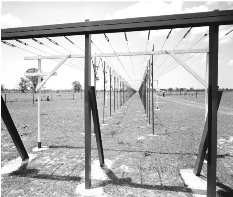
Figure 33. View looking along the E-W arm of the Mills Cross, showing the three major support posts at the end of the arm to which the tensioned wires above the mesh reflector were attachment, 1954. (Source: ANTF Historic Photographic Archive, 3324-1)
