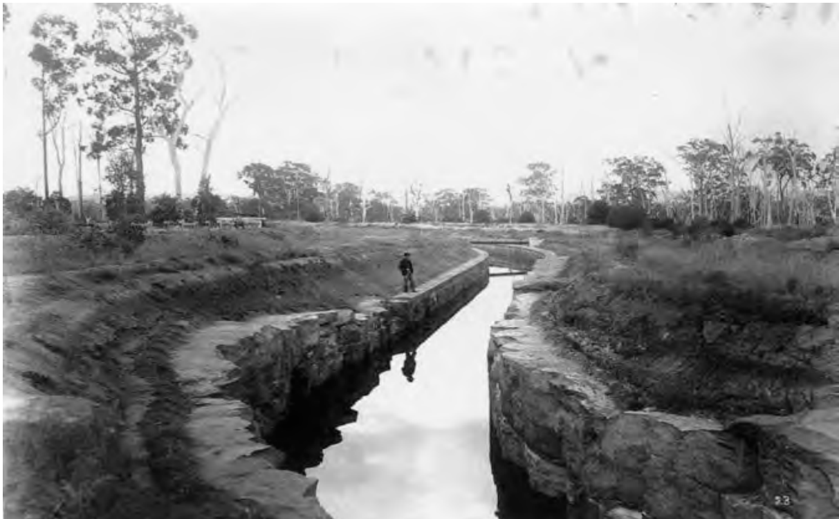
Figure 24: a rock cut and masonry lined section of the Canal c1898 with flume in the background and showing the serpentine nature of the Canal system 2
