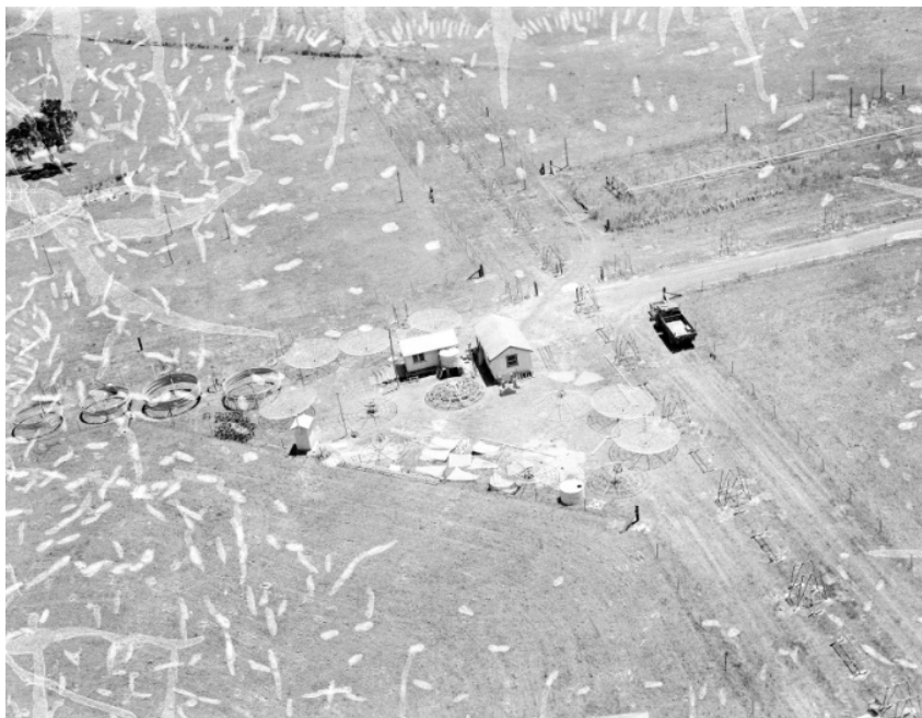
Figure 36. Aerial photograph showing the Chris Cross under construction (but unfortunately not too clearly as the negatives are badly degraded). However, this photograph shows the construction huts at the centre of the array, formwork used when constructing the antennas, and a number of completed antennas. Also visible are examples of the initial framework for each of the antenna mounts. 1956 (Source: ANTF Historic Photographic Archive, B5042-3)
