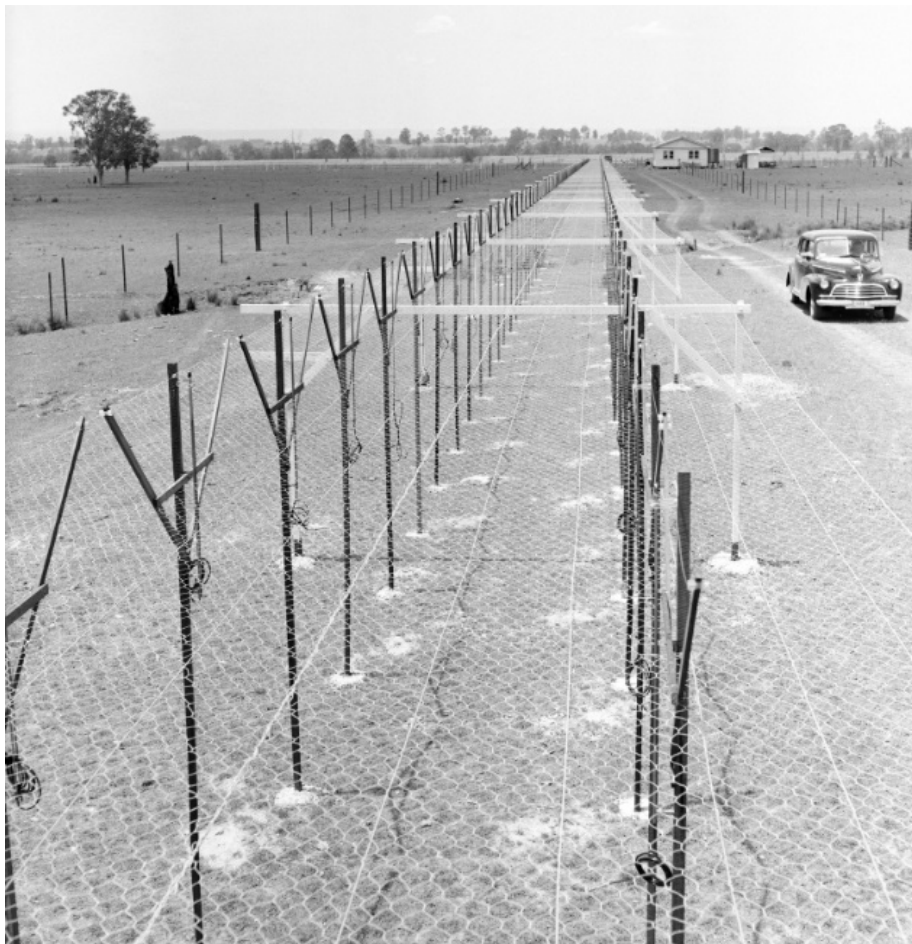
Figure 31. Antenna - General view of strain posts, reflector and dipoles from Eastern end at Fleurs Array, 1954. (Source: ANTF Historic Photographic Archive, 3234-2)
