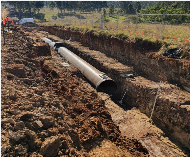
Figure ES7 Trenched pipeline construction with benching
