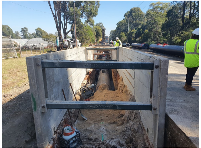
Figure ES8 Trenched pipeline construction with shoring in constrained contexts
