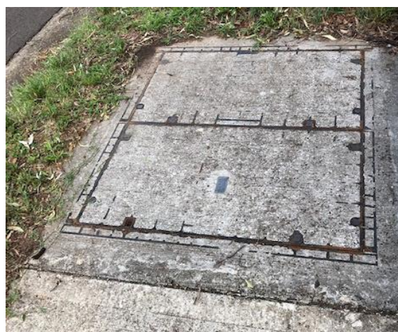
Figure 4-13 Covered sensor box pit
