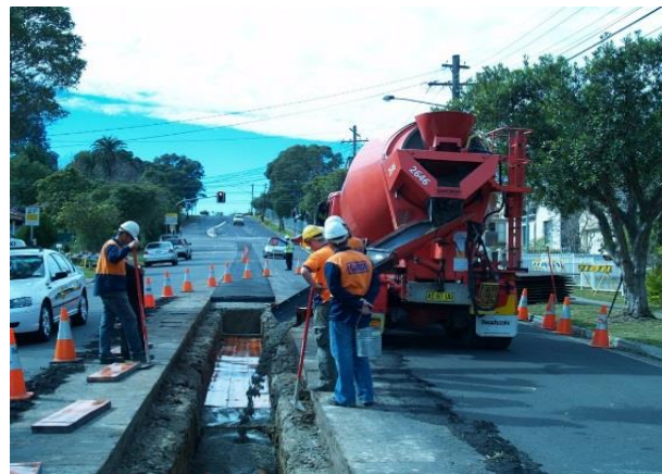
Figure 4-23 Backfilling of a trench
