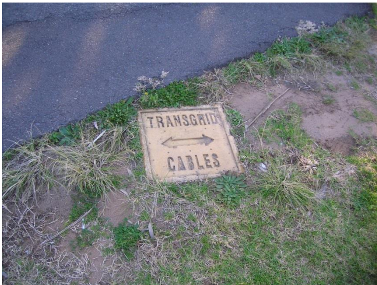
Figure 4-24 Example of a flush marker
