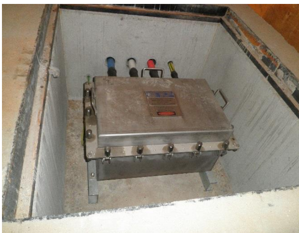
Figure 4-12 Typical link box pit
