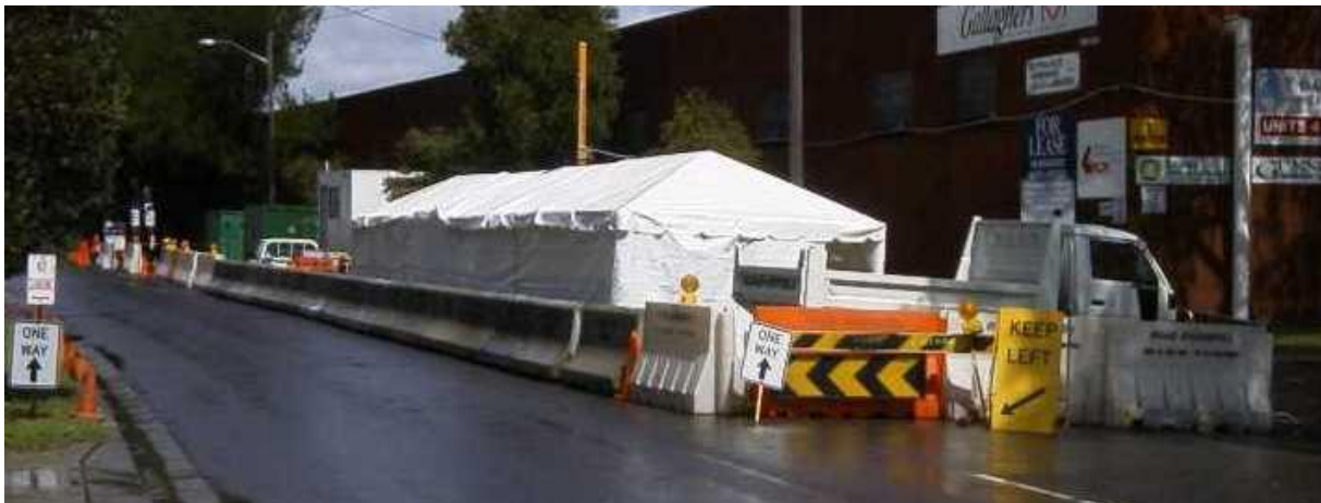
Figure 4-27 Example of cable jointing works occurring under cover
