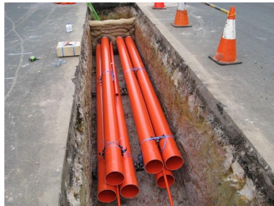
Figure 4-8 Typical double circuit trefoil conduit arrangement
