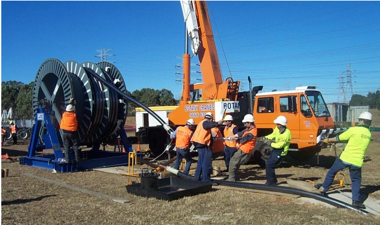
Figure 4-26 Cable pulling
