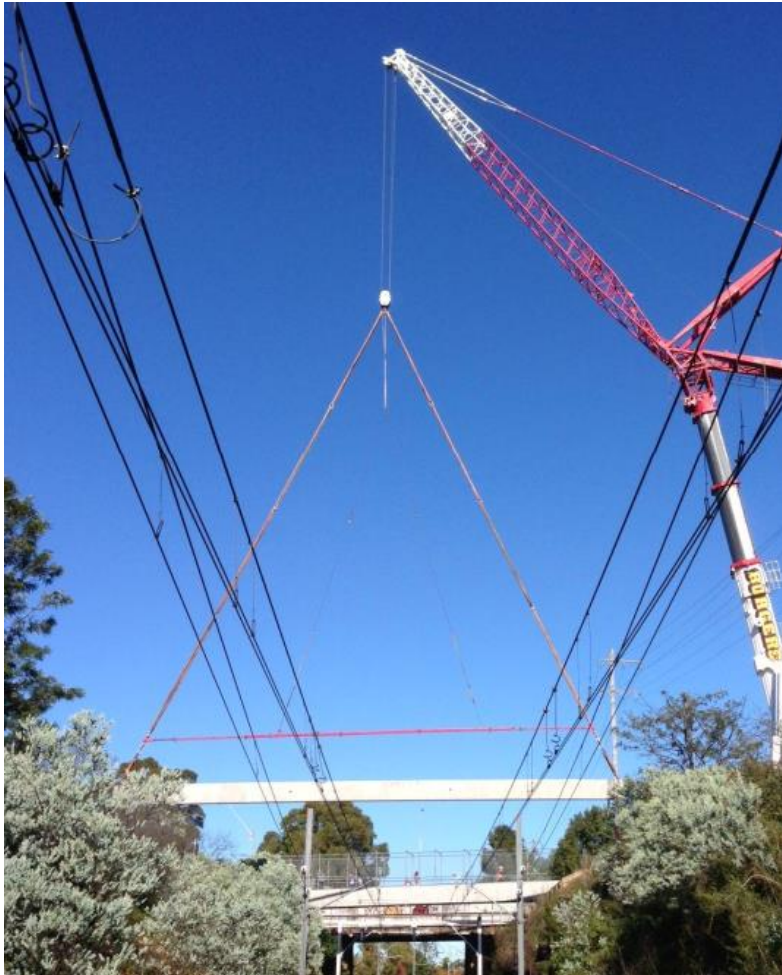
Figure 4-28 Example of a cable bridge being lifted into place as part of TransGrid's Holroyd to Rookwood project
