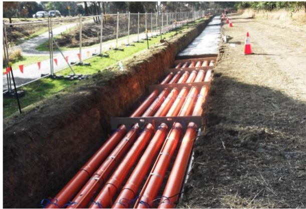
Figure 4-7 Typical double circuit flat conduit arrangement
