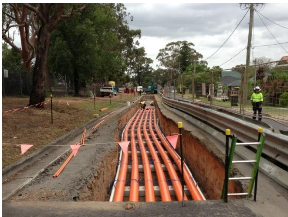
Figure 4-22 Conduit installation within a trench in the roadway
