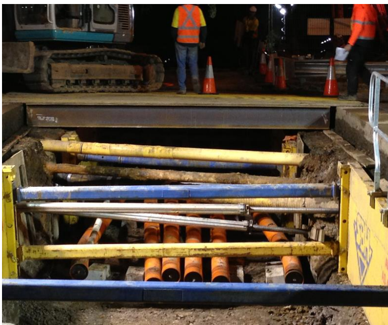
Figure 4-21 Typical arrangement with transmission cable conduits (orange pipes) installed below other services
