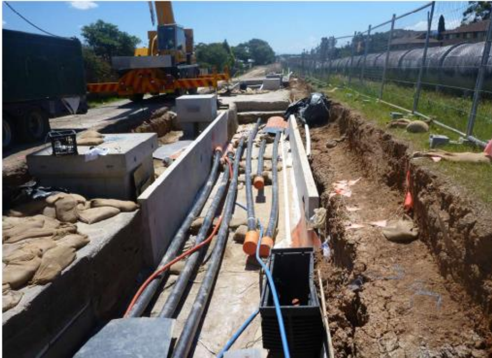
Figure 4-25 Joint bay establishment with link and sensor boxes to the left
