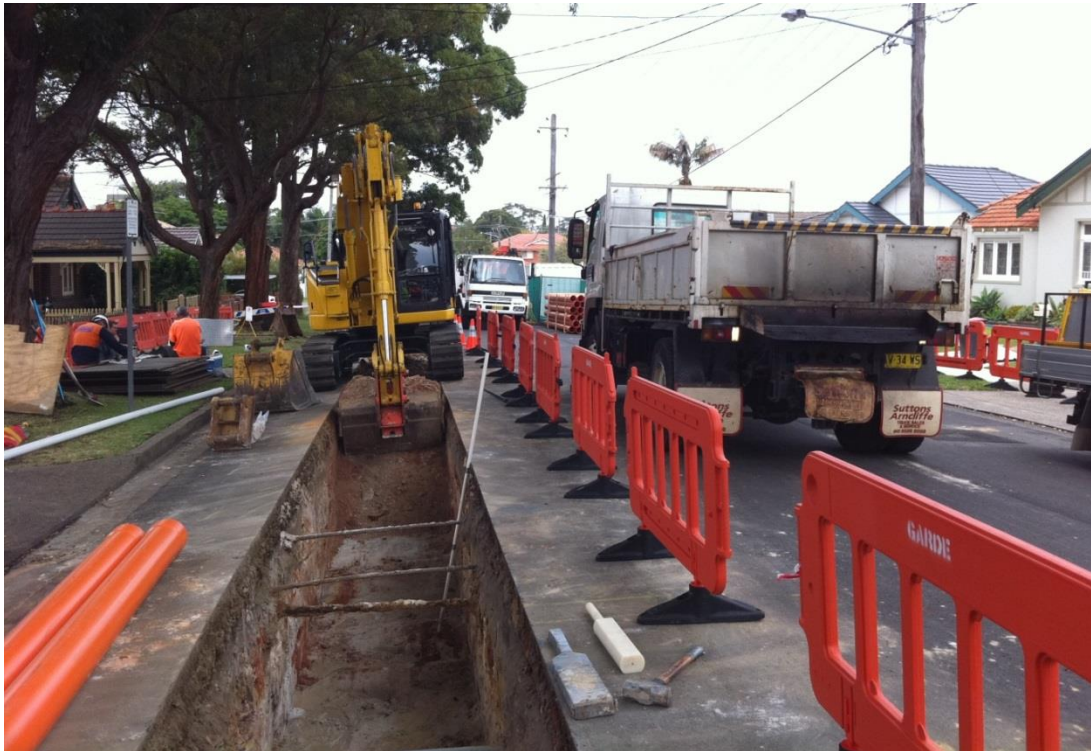
Figure 4-19 Example of trenching within a two lane roadway
