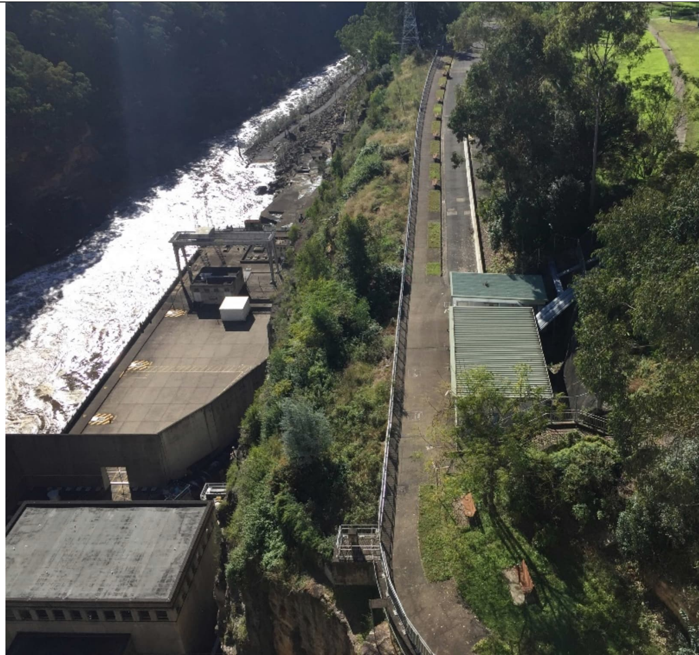
Photograph 3.01 – Looking down onto the electrical building- (large building in foreground) which contains electrical switch boards and a second small building (behind the electrical building), the smaller building reportedly contains a back up power generator. Anecdotal evidence indicates that a 300-400 litre above ground diesel tank is located within the smaller building. There are no plans to disturb these structures during proposed construction works.
