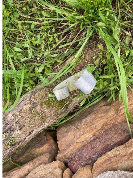
Figure 4-36: Metal bracket nailed into a timber beam.
