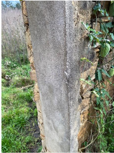
Figure 4-25: Example of lime wash on the interior walls and doorways.
