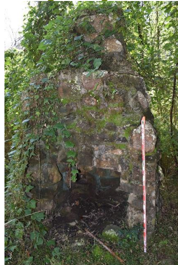
Figure 4-6: The chimney structure with scale (1.3 m).
