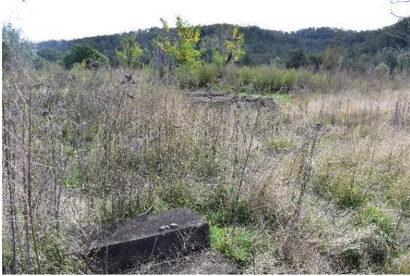
Figure 4-58: View of former structure foundations, facing west.
