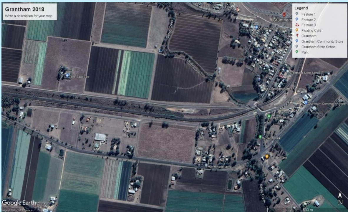
Figure 7 - Aerial photograph of Grantham, Queensland in 2018, after the flood and land swap program, showing partial removal of dwellings from the floodplain (source: Google Earth).
