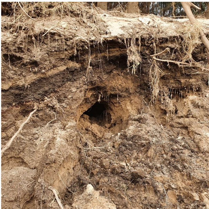
Image 2. Evidence of piping in riverbank downstream of North Richmond
