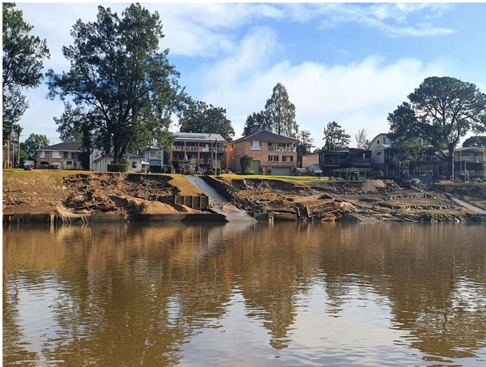
Image 8. Riverbank in the Ebenezer area. There has been significant erosion adjacent to built structures on un-vegetated banks.
