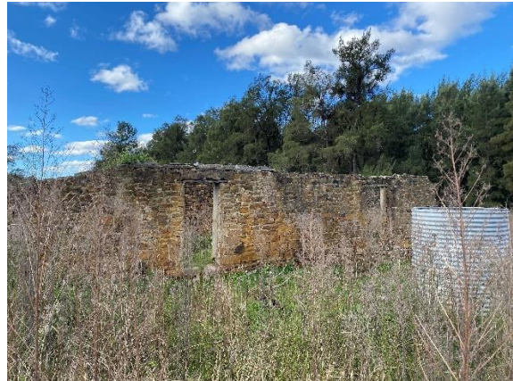
Figure 4-32: View of the tank and southern wall, facing north.
