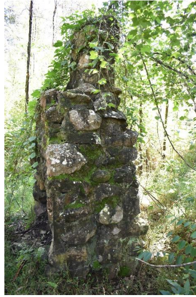
Figure 4-2: Side view of the stone chimney, facing north.
