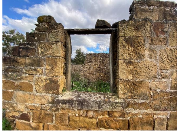
Figure 4-18: Example of a window with timber and sandstone lintels.
