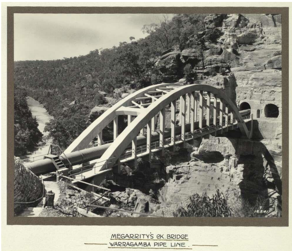
Figure 3-21: Photograph of Megarrity's Bridge, c. 1941. (Source: NLA, PIC/8732/17 LOC Album 562)
