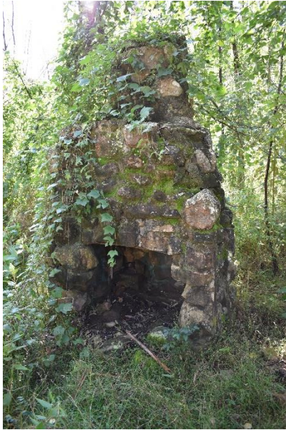
Figure 4-1: Frontal view of the extant stone chimney and fireplace, facing north-east.
