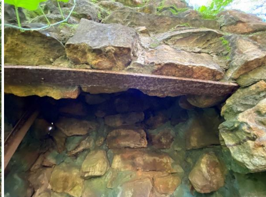
Figure 4-10: Image of the iron lintel above the fireplace.
