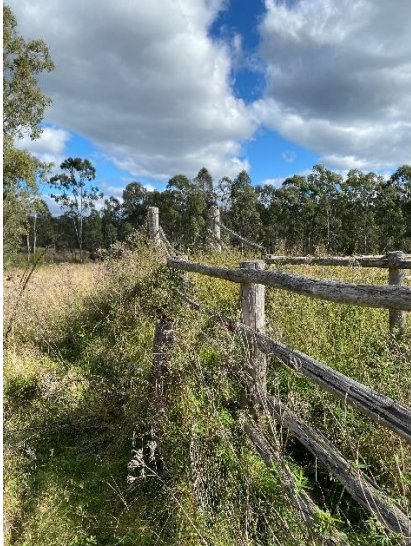
Figure 4-46: Former livestock ramp.
