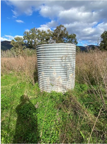
Figure 4-29: Extant corrugated iron water tank.
