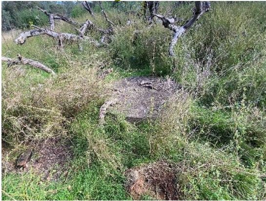
Figure 4-62: Example of a former structure, possible former septic tank.
