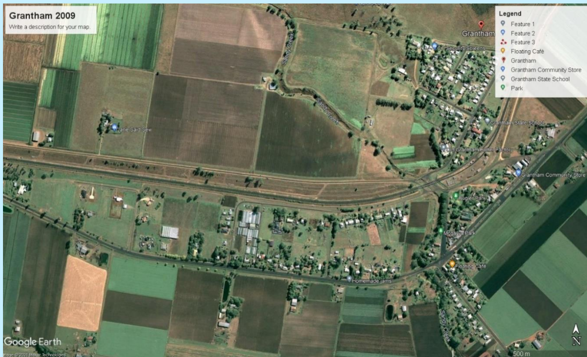
Figure 6 - Aerial photograph of Grantham, Queensland in 2009, prior to the flood and land swap program (source: Google Earth)
