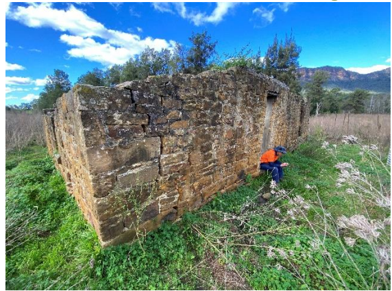
Figure 4-28: View of the southerly wall, facing north east.
