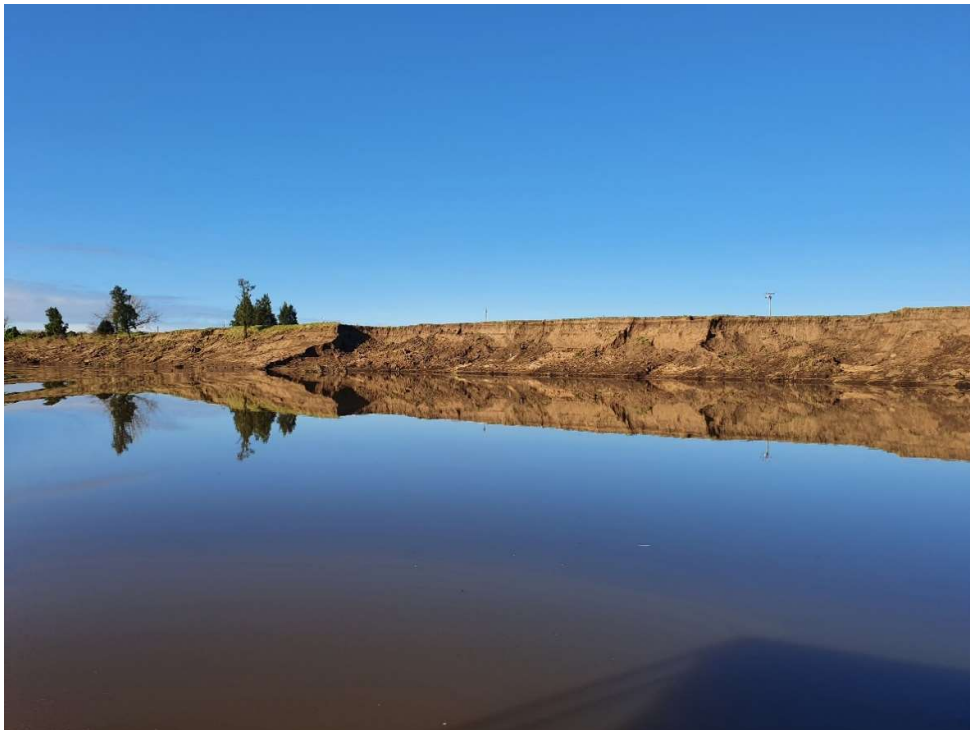
Image 4. Riverbank upstream of Windsor. Note significant erosion from recent flood events.
