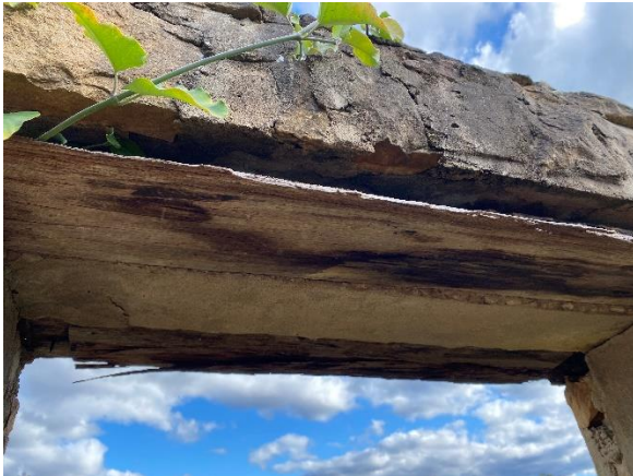
Figure 4-31: Example of the condition of timber lintels.
