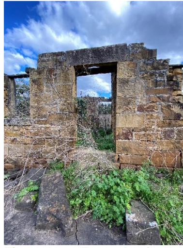
Figure 4-20: Example of a doorway with sandstone and timber lintels.
