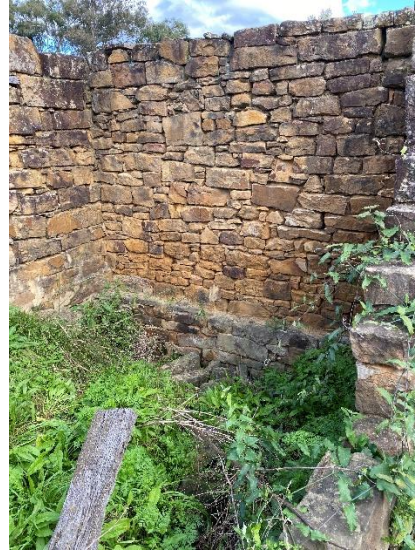
Figure 4-30: View of the third room showing the former floor level and the subfloor level, shown through colour differentiation in the sandstone.
