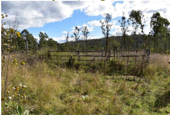
Figure 4-42: Former livestock ramp and yard, with extant fencing, facing west.
