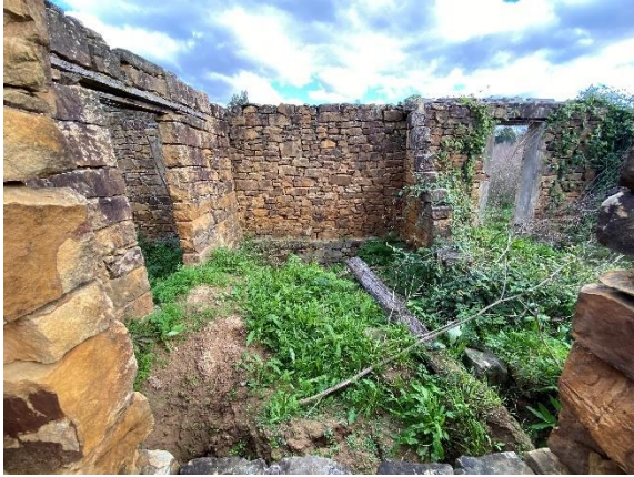
Figure 4-23: View of the two middle rooms, facing south.
