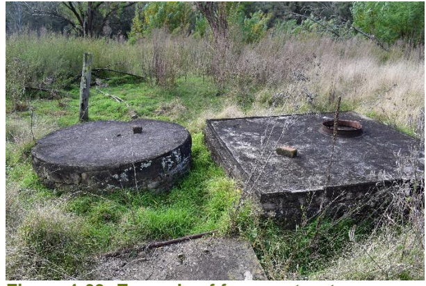
Figure 4-63: Example of former structures, one with stone foundations and one with concrete foundations.
