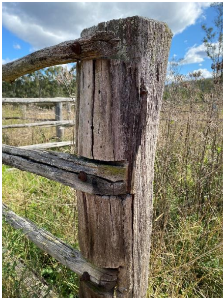
Figure 4-48: Example of bolted rails to end posts at the yard.
