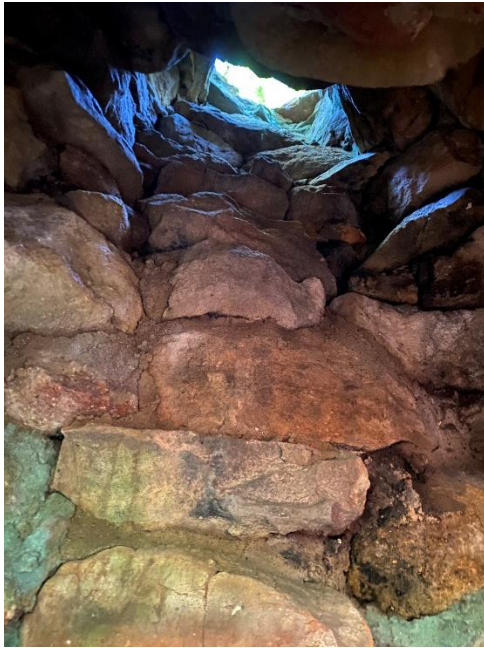
Figure 4-13: View inside the chimney flue.
