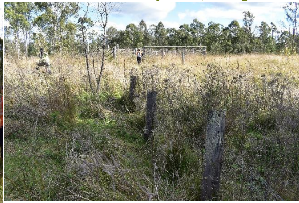
Figure 4-43: View of the livestock ramp and yard, with extant fencing, facing south.
