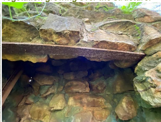
Figure 4-10: Image of the iron lintel above the fireplace.
