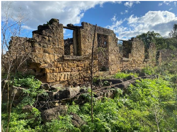
Figure 4-15: View of the northern façade of the stone hut ruins, showing the collapsed veranda and eastern wall.
