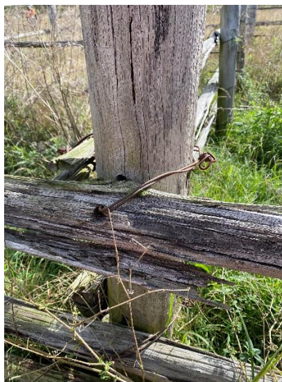
Figure 4-47: Example of the high tensile fencing wire used to tie the rails to the posts at the yard.
