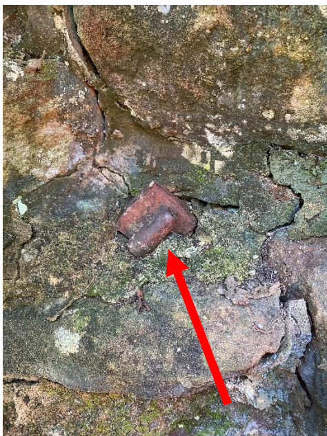
Figure 4-11: Image of one of the steel bolts protruding from the side of the chimney.
