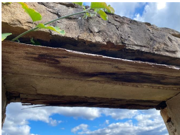
Figure 4-31: Example of the condition of timber lintels.
