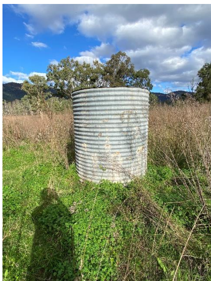
Figure 4-29: Extant corrugated iron water tank.
