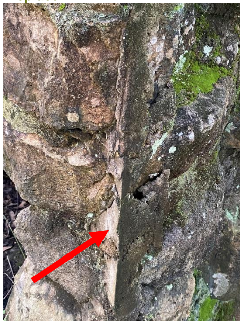
Figure 4-12: Image of one of the external sides of the chimney, showing possible former joint or wall.
