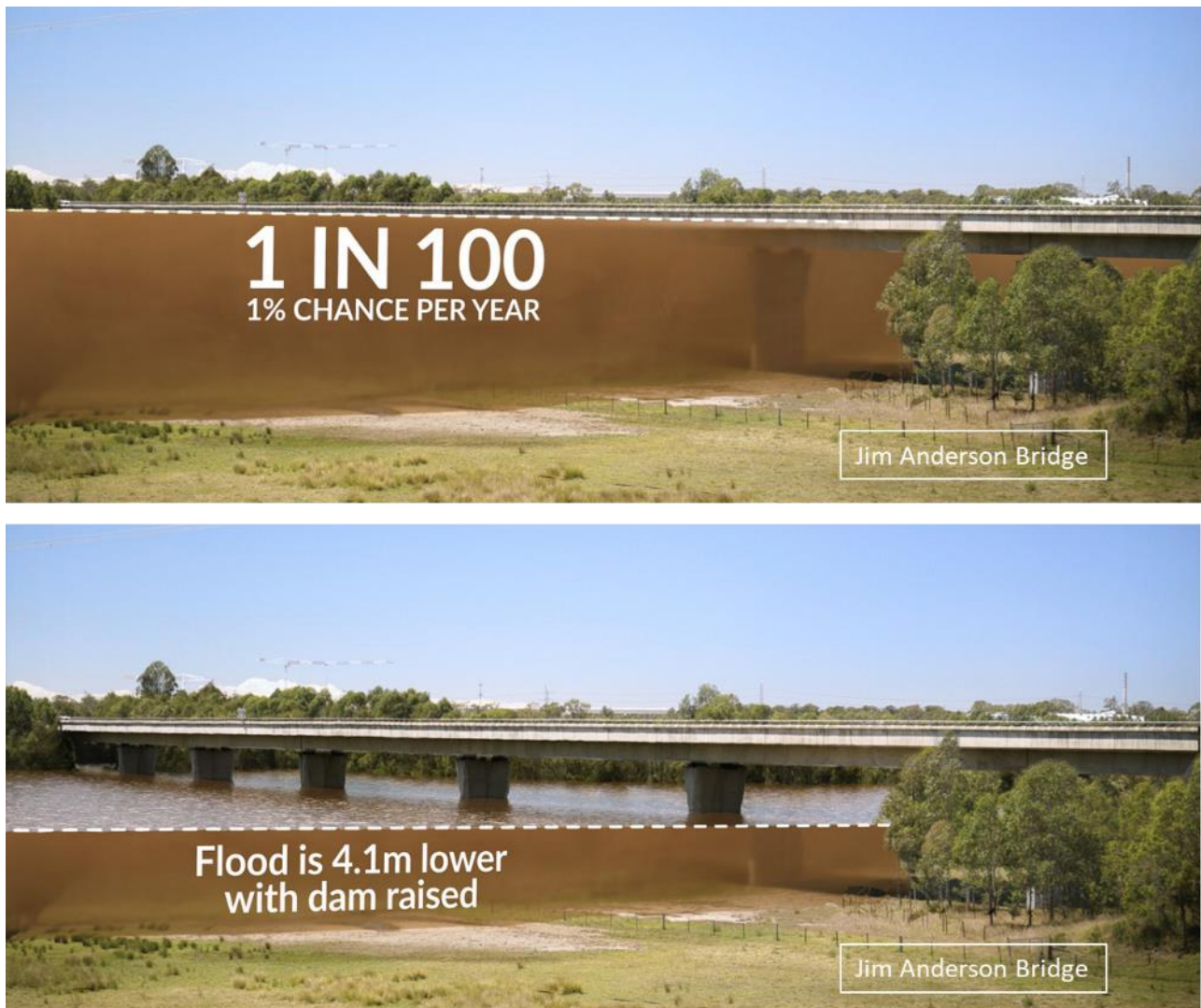
Figure 9 Jim Anderson Bridge (Windsor) 1 in 100 chance in a year flood – without and with raised dam
