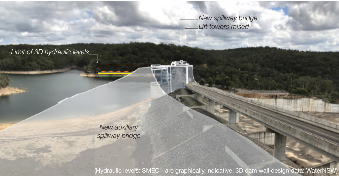
Figure 5-29: Viewpoint 2-1 - Photomontage view looking northwest over the upgraded auxiliary spillway and bridge towards the dam
