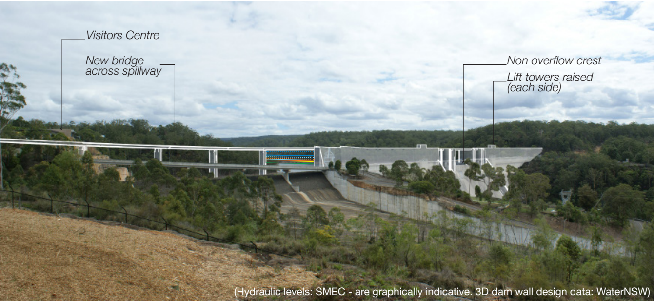
Figure 5-33: Viewpoint 2-3 - Photomontage view showing raised dam wall and bridge over spillway
