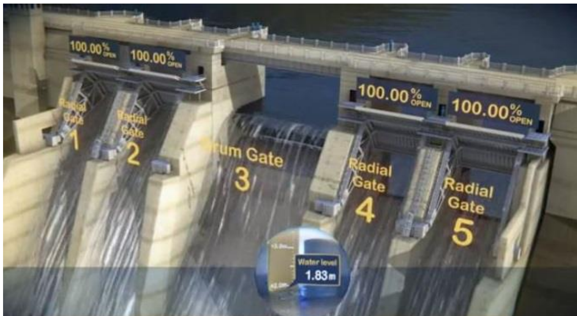
Figure 3-12 How the gates on Warragamba Dam work (Source: WaterNSW Website)
