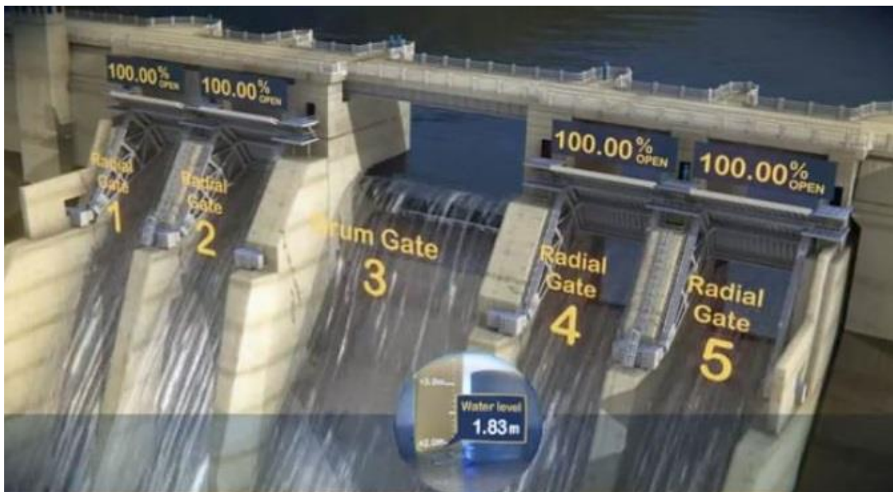
How the gates on Warragamba Dam work (Source: WaterNSW Website)
