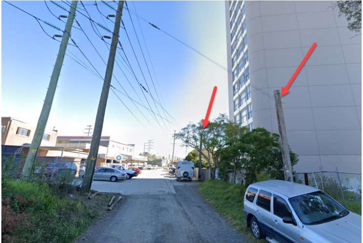
Figure 3.88: Existing Ausgrid high voltage aerials and stay poles
