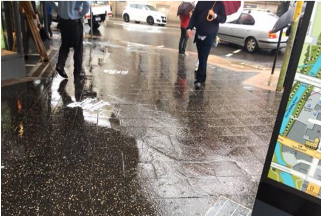
Figure 19 Ponding in footpath sag – north-west corner of George/Church Street intersection
