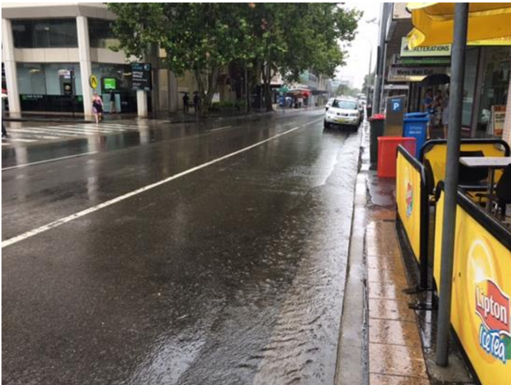
Figure 18 Flow in gutter along the southern side of Macquarie Street looking east towards Horwood Place intersection (Source: Transport for NSW)
