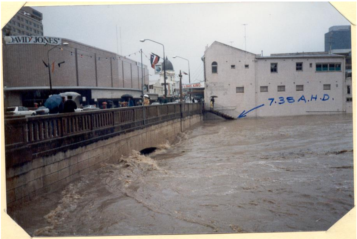
Figure 12 Lennox Bridge (upstream face – western side), 30 April 1988 (Source - CoP)
