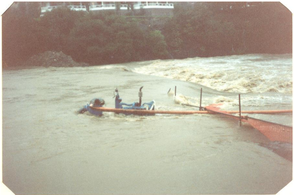
Figure 10 Overtopping of Charles Street Weir - date unknown (Source - CoP)
