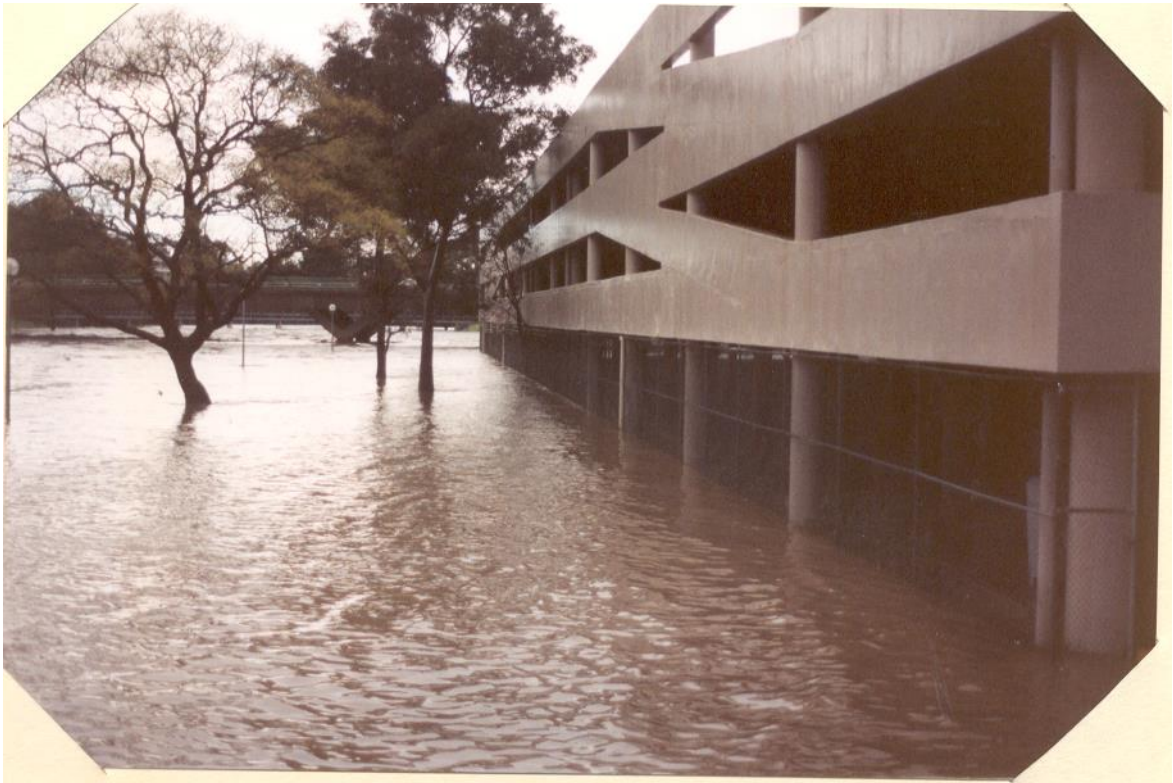
Figure 8 Riverbank Car Park facing east towards Wilde Avenue Bridge – 1988 (Source - CoP)
