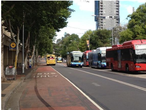
Kerbside bus lanes in Argyle Street, Parramatta at the Westfield shopping centre as part of the T-way network
