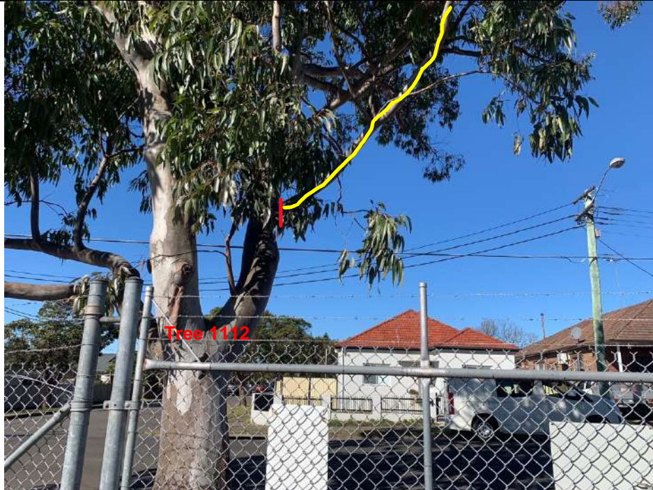
Image 14: Looking towards tree 1112, showing required canopy pruning. The 120mm second order branch to the West at 3m above ground is to be removed. The branch has been marked yellow and the final pruning cut has been marked red. The pruning will result in the removal of less than 5% of the overall live canopy.
