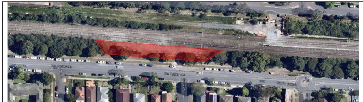
Image 10: The Boulevard works area from JHLOR
