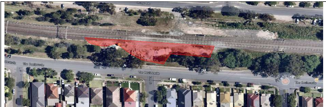
Image 13: The Boulevard works area from JHLOR
