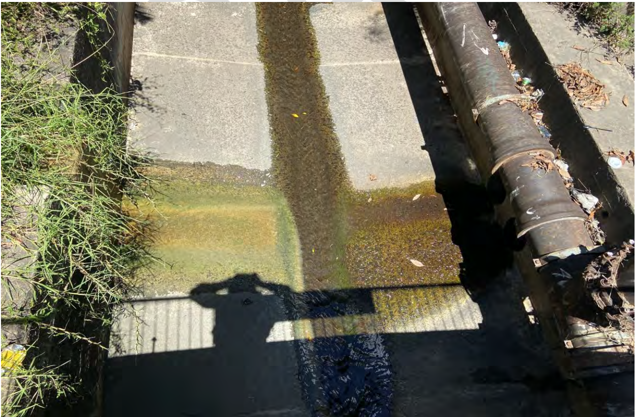
Photograph 4. Minor stormwater in-flow observed from both discharge points WP2-DP1 and WP2-DP2 which were located within the rail corridor and immediately upstream / south from WP2 during the monitoring event – 09.02.2022
