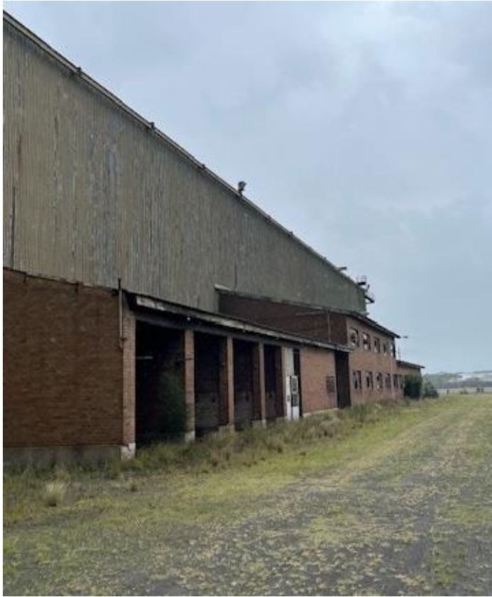
Photograph 12: Eastern exterior of the Roll Shop
