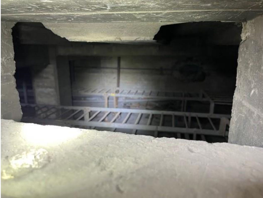
Photograph 17: The confined space via the entrances.
