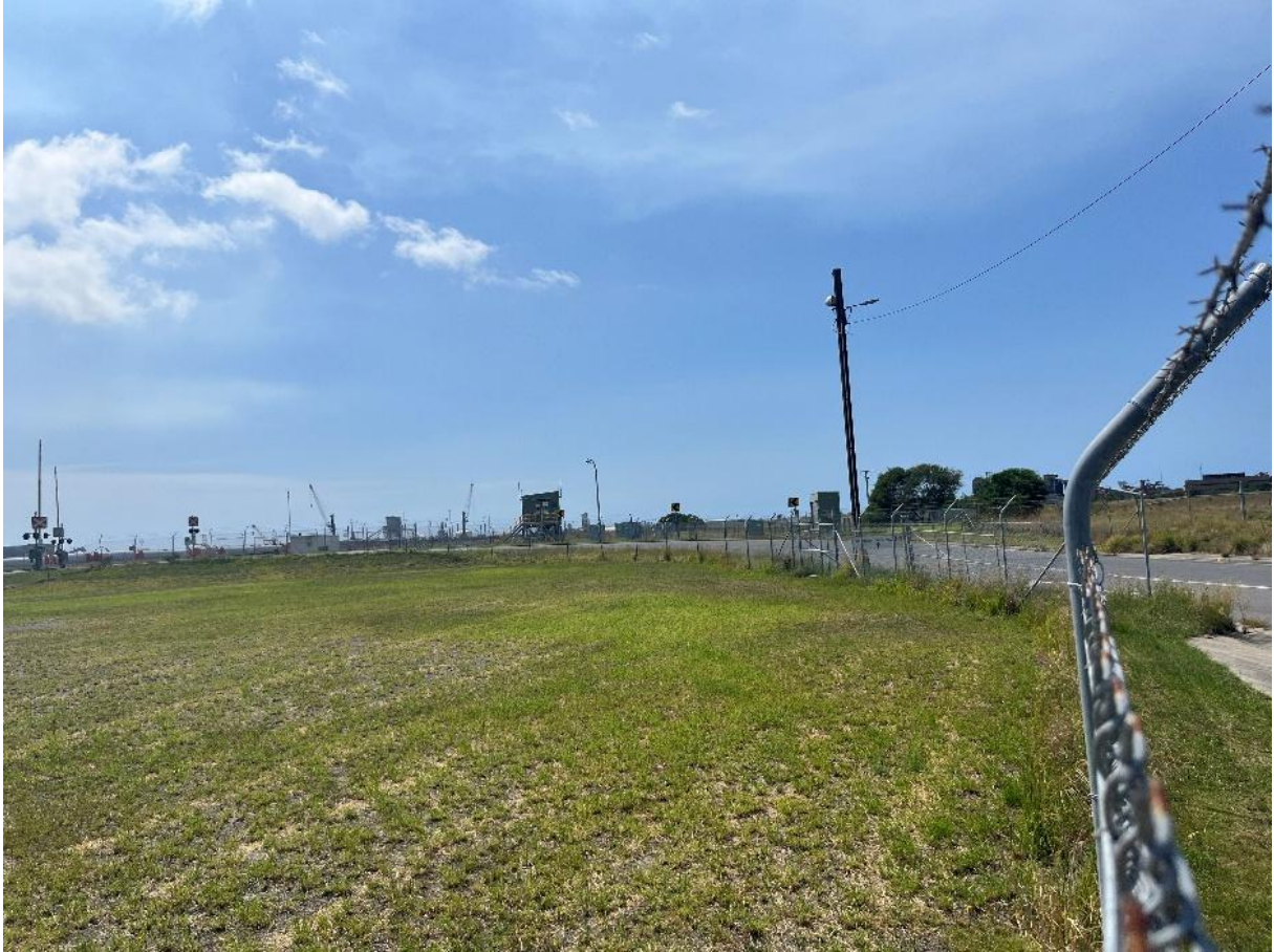
Photograph 1: Proposed additional access / hardstand area. Taken from Steel Works Road facing north.
