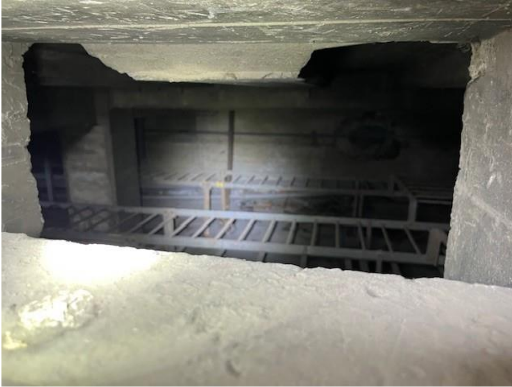
Photograph 17: The confined space via the entrances.
