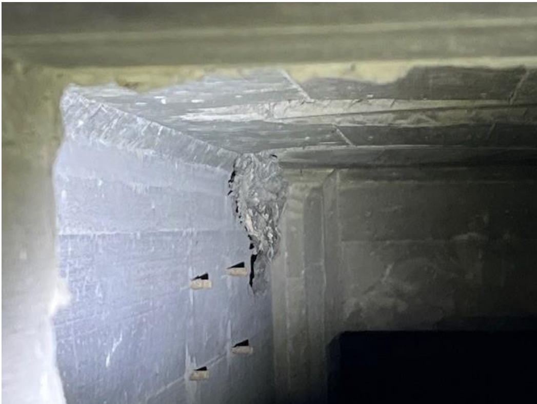
Photograph 18: The confined space via the entrances
