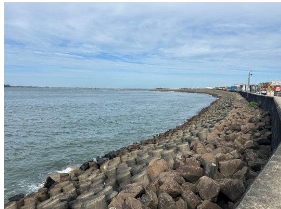
Plate 2 View southwest of southern revetment wall (Source: AECOM, 2025).
