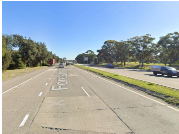
Figure 3-2 Foreshore Road, west of Penrhyn Road (looking west) Source: Google Maps, 2024
