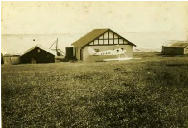
PHOTOGRAPH 4-4 NEWLY CONSTRUCTED CARGO SHED WITH SEAPLANE AT REAR, 1931 (LHI MUSEUM)
