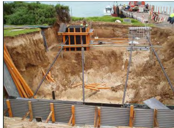
PHOTOGRAPH 5-3 JETTY WORKS AND , 2007. EXTENSIVE EXCAVATION WITHIN AREA OF FORMER SHEDS (LHIB)
