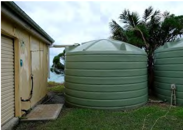
PHOTOGRAPH 4-44 TANKS TO NORTH OF OV SHED (ADJACENT TO PROPOSED REMOVED ADDITION)
