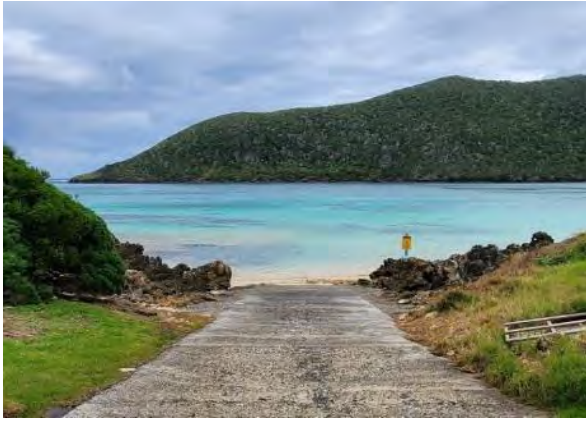
PHOTOGRAPH 4-24 BOAT RAMP, FACING NORTHWEST
