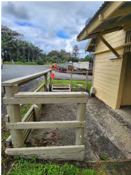
PHOTOGRAPH 4-32 CARGO SHED EAST ENTRANCE WITH TIMBER STEPS, RAILS AND RETAINING WALL
