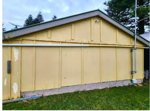
PHOTOGRAPH 4-39 OV SHED, WEST ELEVATION
