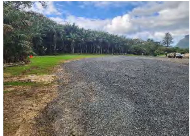
PHOTOGRAPH 4-23 FACING SOUTHEAST ACROSS HARDSTAND
