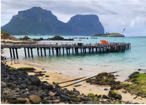
PHOTOGRAPH 4-46 JETTY, VIEW FROM NORTH
