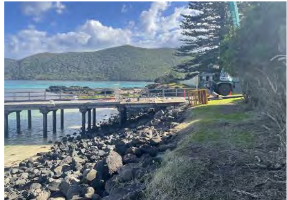
PHOTOGRAPH 4-49 JETTY AT LAND JUNCTION, FACING NORTH
