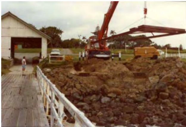
PHOTOGRAPH 5-2 JETTY WORKS, 1982. NOTE MAJOR SEAWALL AND FORESHORE MODIFICATION (LHIB)
