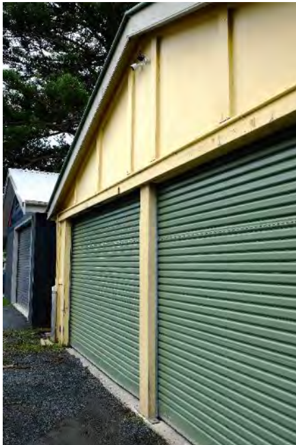
PHOTOGRAPH 4-40 DETAIL OF EAST ELEVATION
