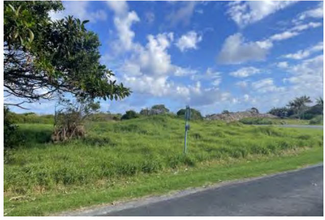
PHOTOGRAPH 4-59 PROPOSED FUEL BOWSER SITE, LOOKING NORTHWEST – WMF ENTRANCE IN BACKGROUND
