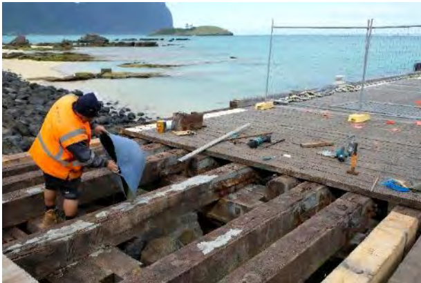
PHOTOGRAPH 4-48 ROTTEN JOIST REPAIR IN PROGRESS, JULY 2025
