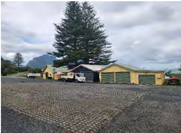
PHOTOGRAPH 4-22 FACING WEST TOWARDS SHEDS (OV SHED ON FAR RIGHT)
