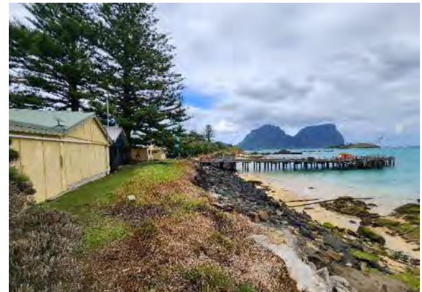
PHOTOGRAPH 4-45 VIEW SOUTH - NOTE RAILS AT SHORELINE INDICATING LOCATION OF ORIGINAL OV BOAT RAMP
