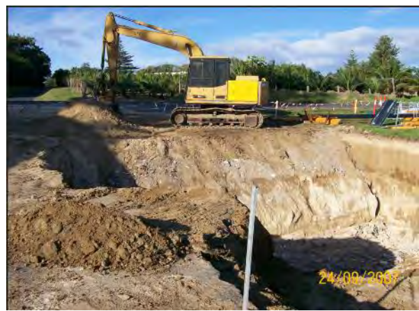
PHOTOGRAPH 5-5 JETTY AND FORESHORE STABILISATION WORKS, 2007 (LHIB)
