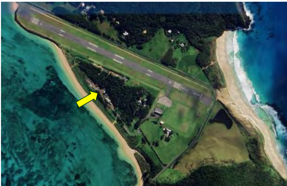
FIGURE 4-5 EVOLUTION OF SOUTHERN PART OF LHI. WMF INDICATED BY ARROW (GOOGLE EARTH PRO, 2025)
