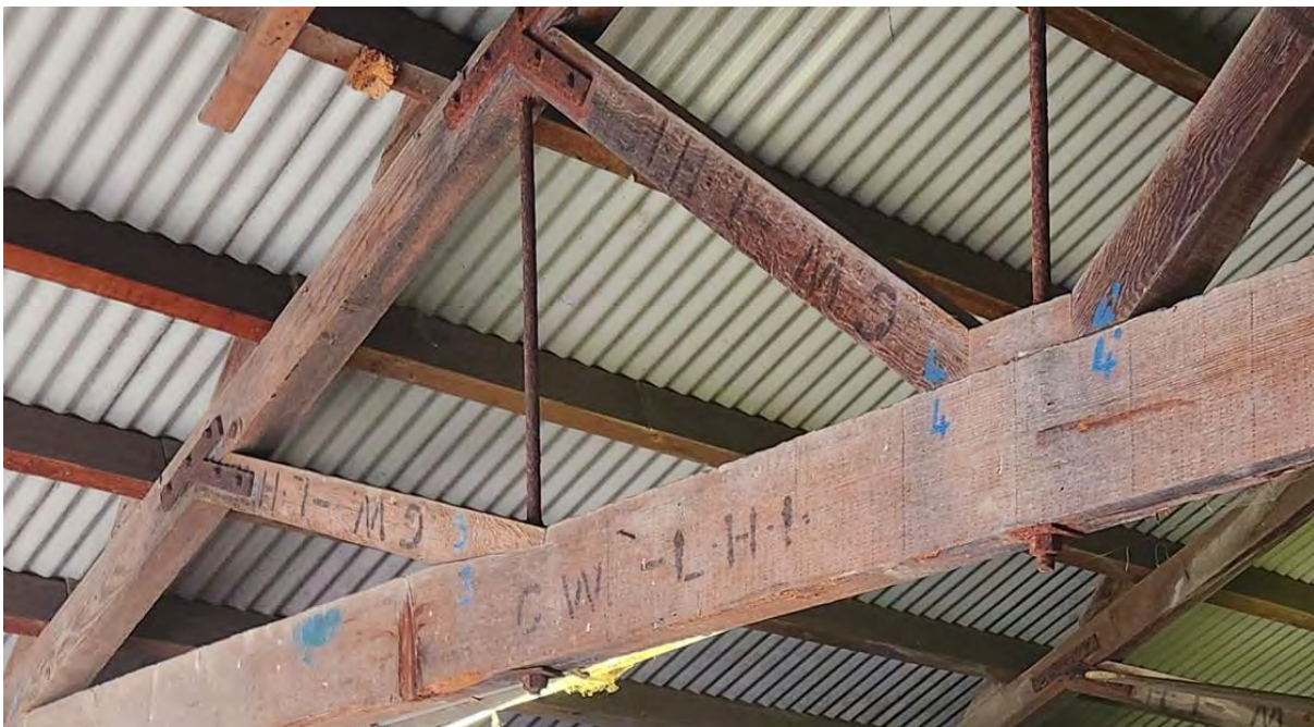
PHOTOGRAPH 7-1 ORIGINAL ROOF TRUSS MEMBERS WITH 'GW - LHI'
