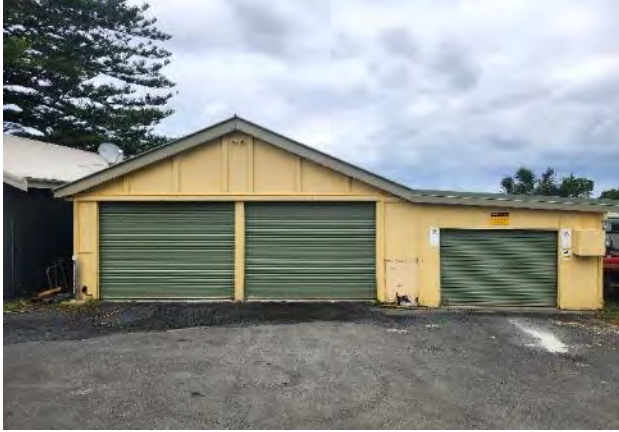
PHOTOGRAPH 4-38 OV SHED, EAST ELEVATION
