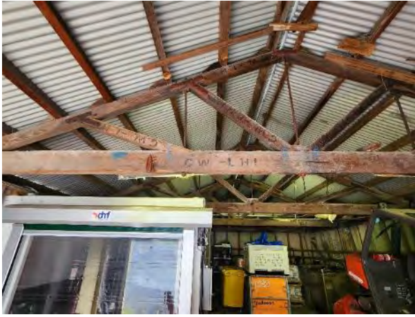
PHOTOGRAPH 4-42 ORIGINAL ROOF TRUSS STRUCTURE, NOTE 'GW LHI' - GEORGE WILSON, LHI
