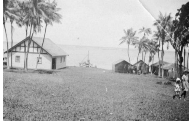
PHOTOGRAPH 4-7 CARGO SHED FROM THE NORTHEAST, C1930S (SOURCE: MUSECAPE PTY LTD, ASSESSMENT OF HERITAGE IMPACT OF DECK AT WESTERN END OF THE FORMER CARGO SHED, LHI MUSEUM, IMG127)
