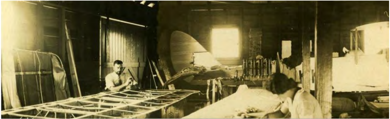
PHOTOGRAPH 4-3 FRANCIS CHICHESTER REPAIRING SEA PLANE WING IN THE CARGO SHED, 1931 (SOURCE: LHI MUSEUM)
