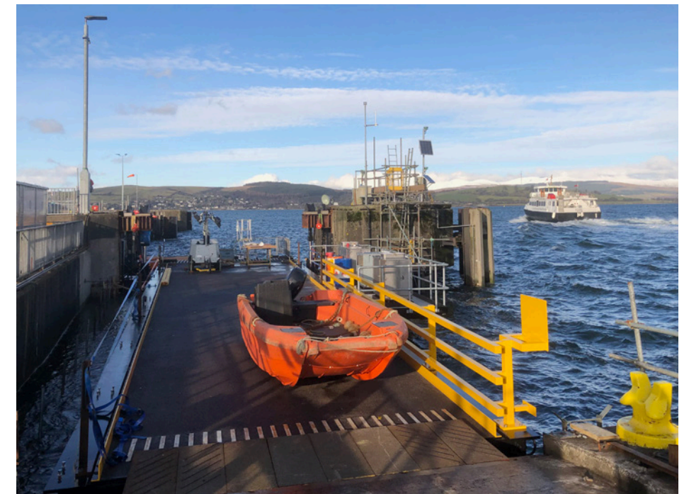
Figure 48: Example of a Linkspan (RoRo)
