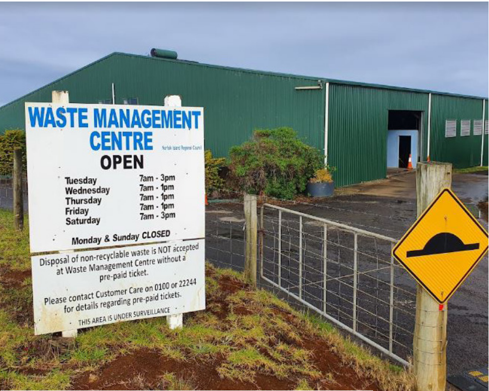
MAIN ENTRANCE - OPERATION HOURS
