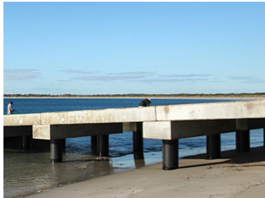
Figure 47: Example of a Fixed Piled Ramp (RoRo)
