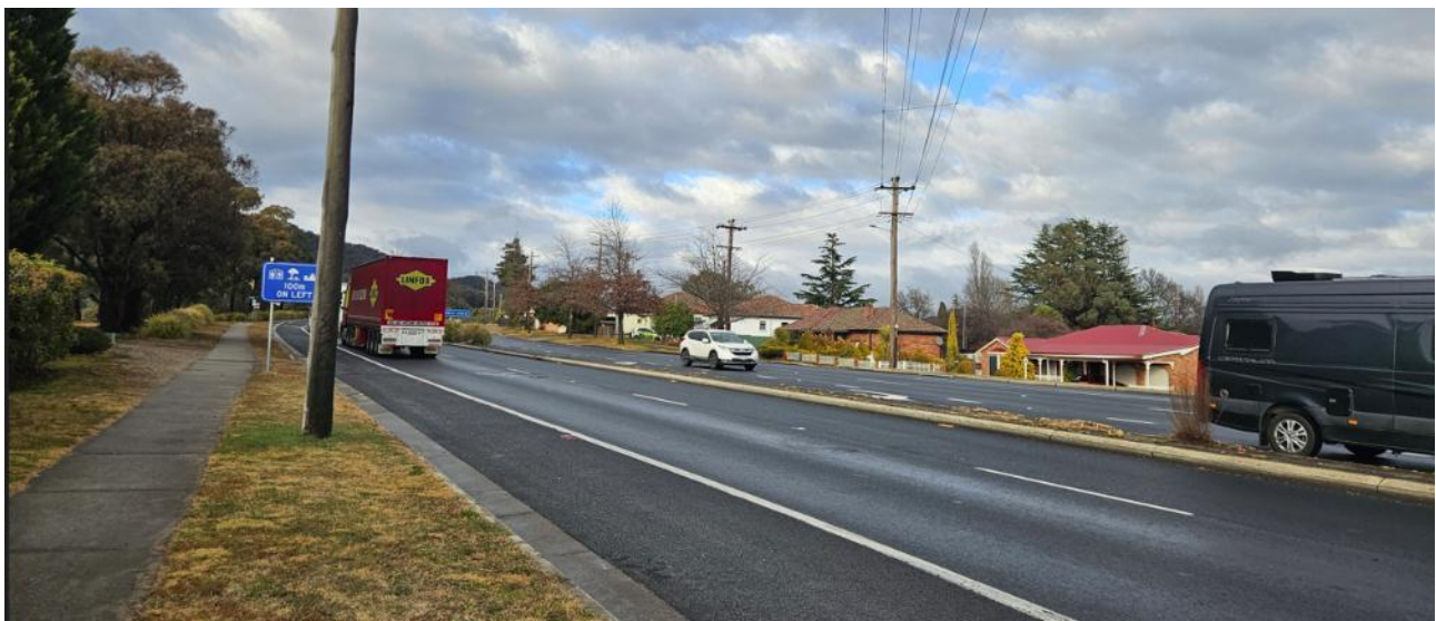
Photograph 3.3 Great Western Highway (view from Bayonet Street)
