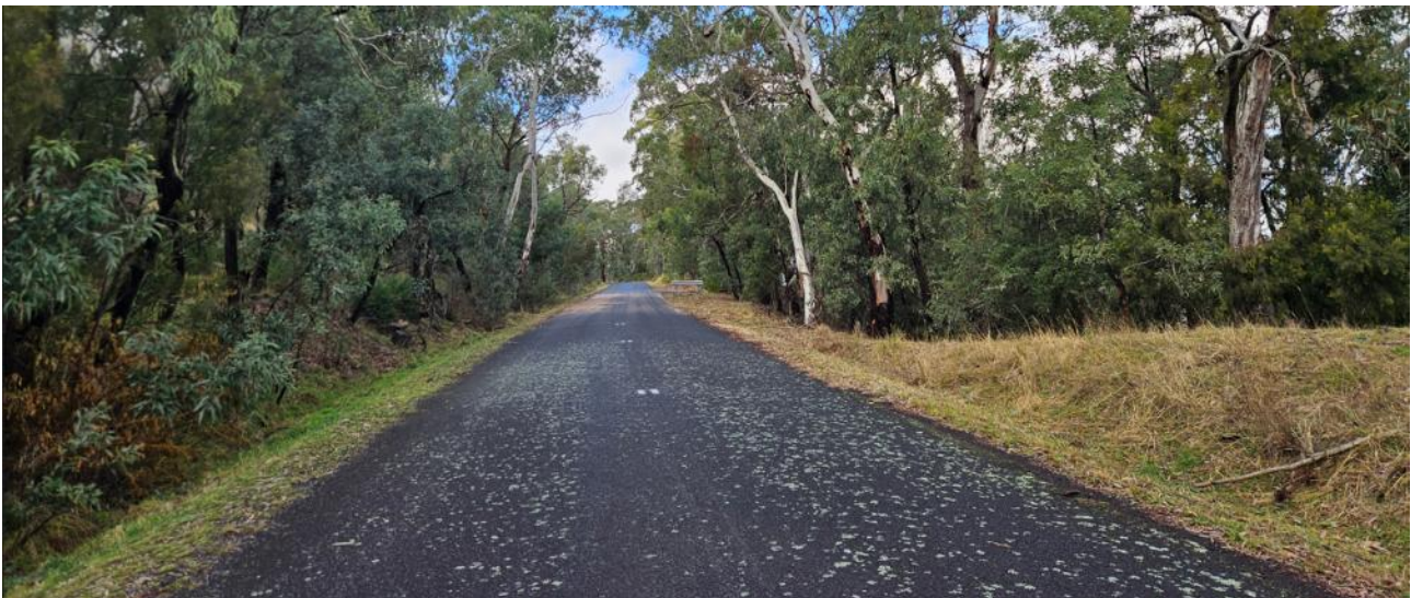
Photograph 3.5 Sir Thomas Mitchell Drive (view from north)
