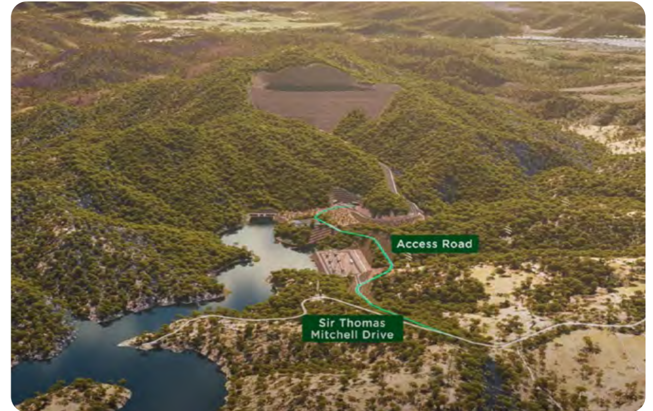
Above: Visualisation of new site access road to be built off Sir Thomas Mitchell Dr, also showing switchyard location. (Source: EnergyAustralia)
