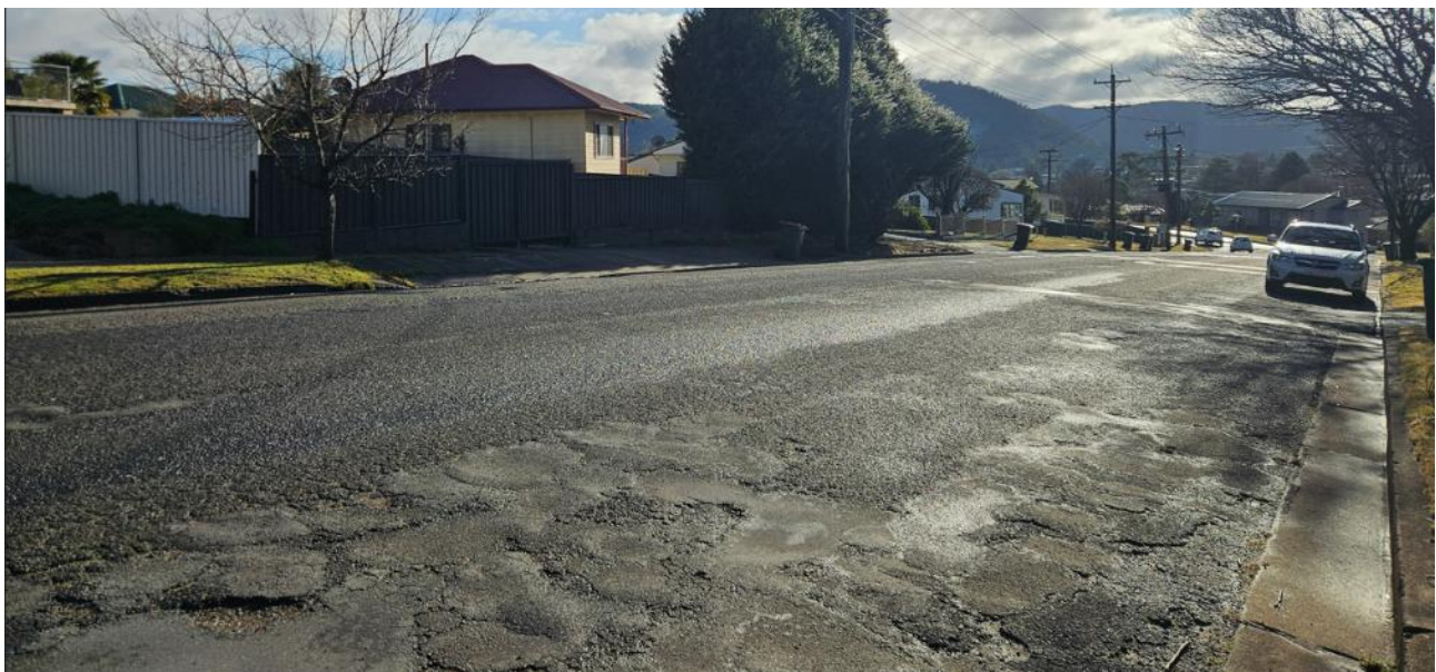
Photograph 3.7 Bayonet Street (view from Great Western Highway)
