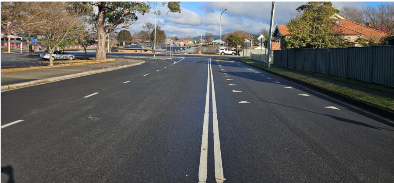
Photograph 3.11 Bent Street near Lithgow Street (view from east)
