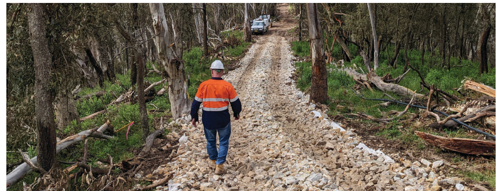
Photograph | Geotechnical investigations access works
