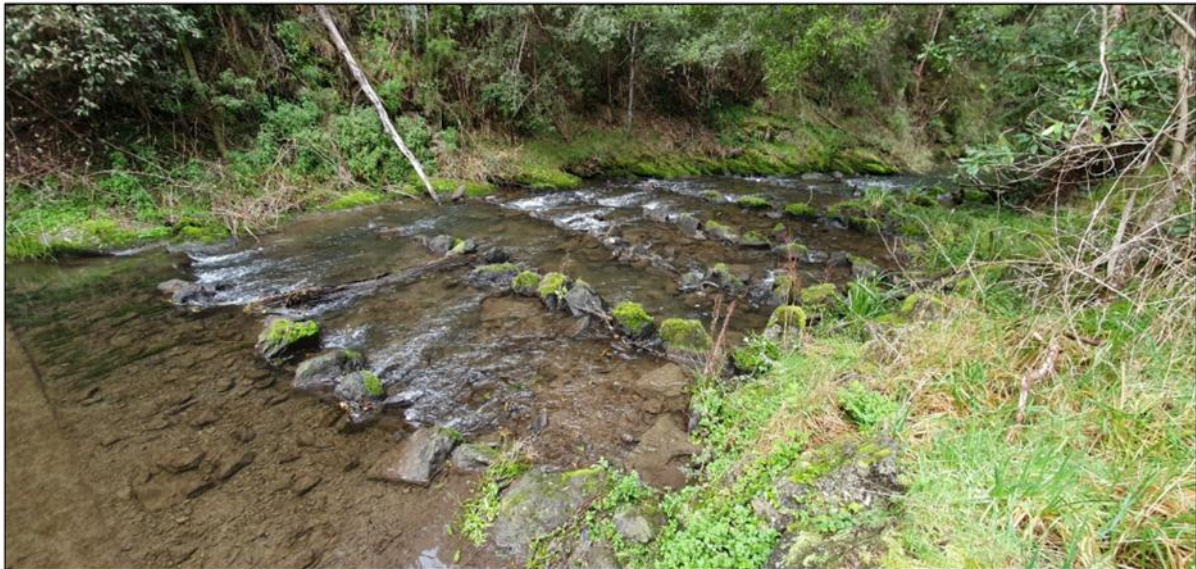
Figure 36: East Barham full-width lateral-ridge rock fishway in temperate Victoria (Stuart, et al., 2024)
