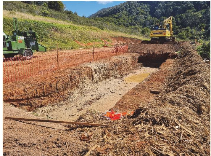
**Image 2: Bruxner Park Rd (sth side) – Establishment of pads and bays for upcoming management of under boring slurry**
