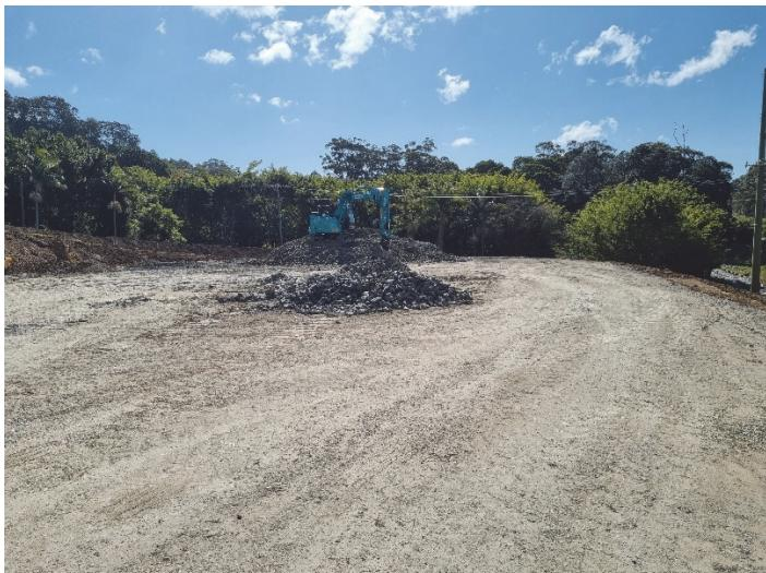
**Image 3: Bruxner Park Rd (nth side) – Establishment of pads for upcoming laydown of utility relocation materials**
