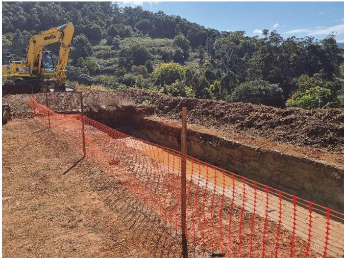
**Image 1: Bruxner Park Rd (sth side) – Establishment of pads and bays for upcoming management of under boring slurry**
