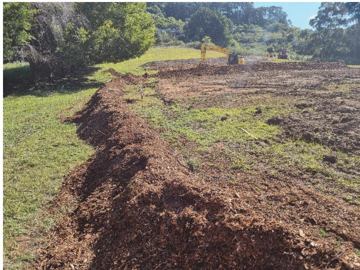
**Image 5:** Bruxner Park Rd (nth side) – Establishment of dewatering bays for future management of under boring slurry
