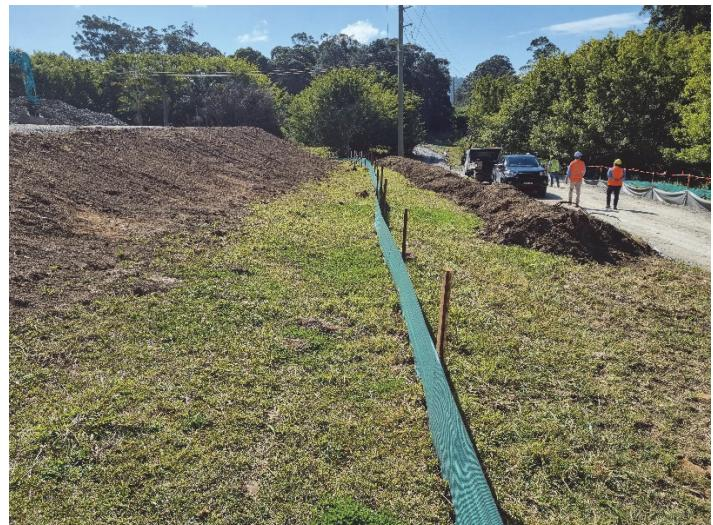
**Image 4: Bruxner Park Rd (nth side) – ErSed controls on downslope side of laydown pad**
