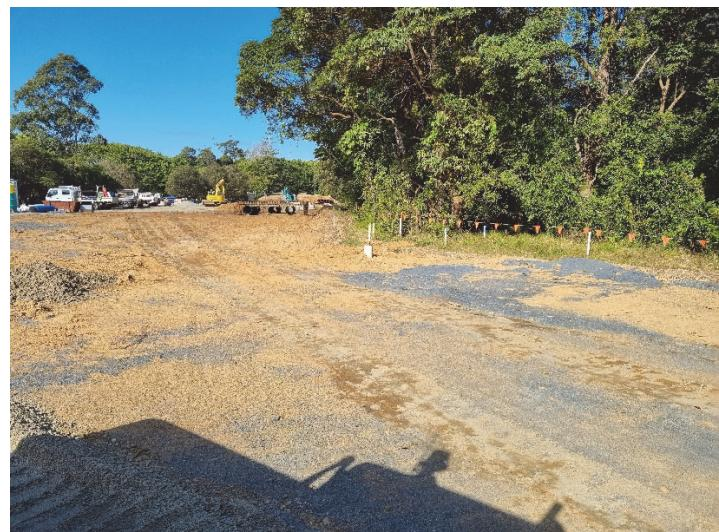
**Image 7:** Opal Blvd utility relocations – site of recent water main installation following backfilling
