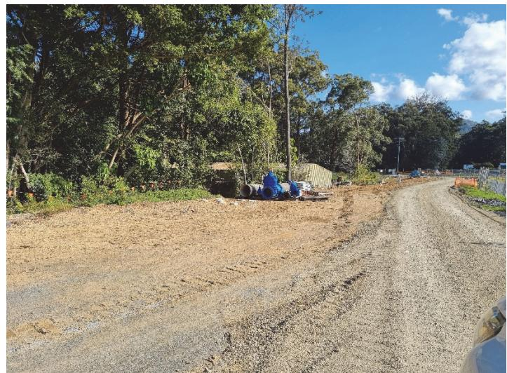
**Image 8:** Opal Blvd utility relocations – site of recent water main installation following backfilling
