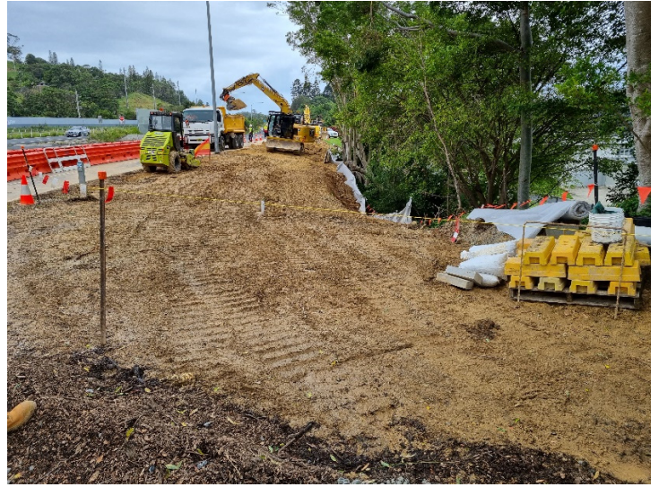
Image 6: Coachmans Close water main relocation (nth side of hill; open trench excavation and installation)
