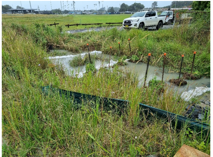
Image 4: Stadium Dr environmental event (frac out). Controls implemented downstream
