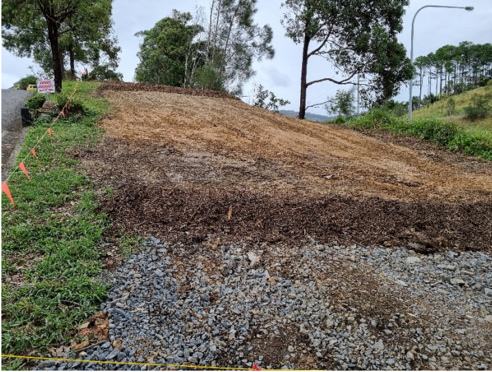
Image 5: Coachmans Close water main relocation (nth side of hill stabilised with gravel material and mulch bunds)
