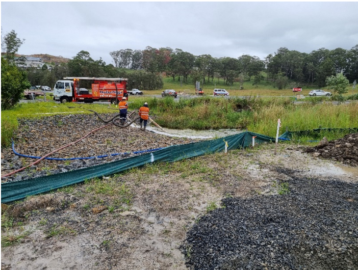
Image 3: Stadium Dr environmental event (frac out). Vacuum truck being used to pump out turbid water
