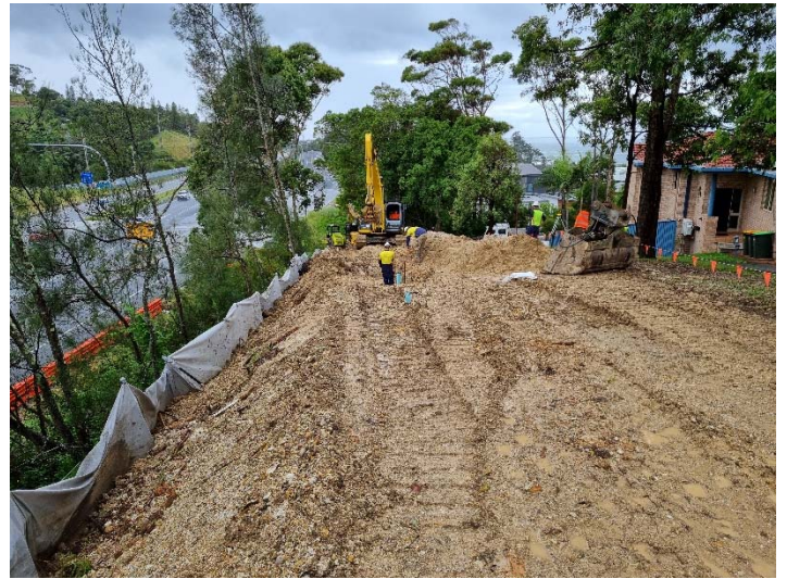
Image 2: Coachmans Close water main relocation (nth side of hill; open trench excavation and installation)
