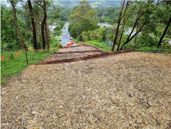
Image 1: Coachmans Close water main relocation (sth side of hill stabilised with gravel material and mulch bunds)
