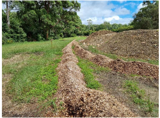
Image 6: Opal Blvd utility relocations (mulch bunds)
