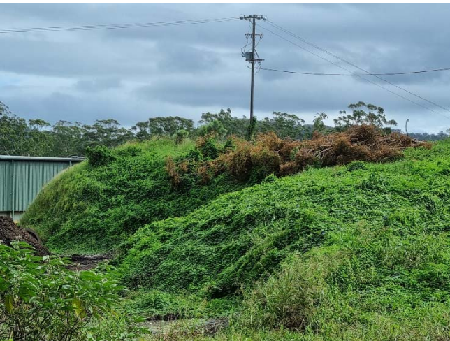
Image 3: Rocky knoll that requires removal for utility install (adjacent Biomass Solutions Ch 10500)
