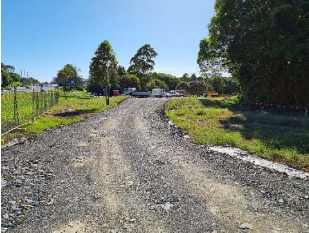
Image 5: Opal Blvd utility relocations (general view of minor ancillary facility)
