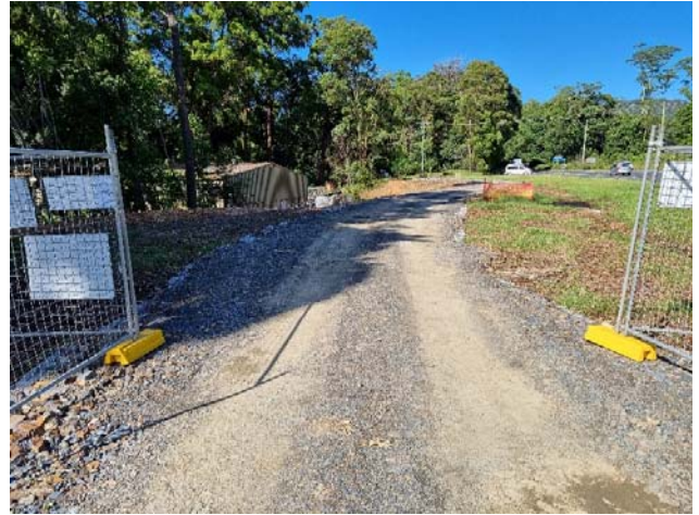
Image 6: Opal Blvd utility relocations (looking south to James Small Dr)
