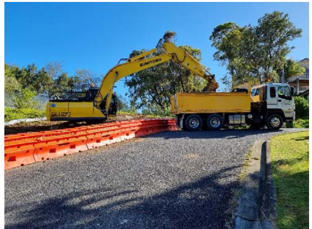
Image 4: Coachmans Close water main relocation (open trench excavation)
