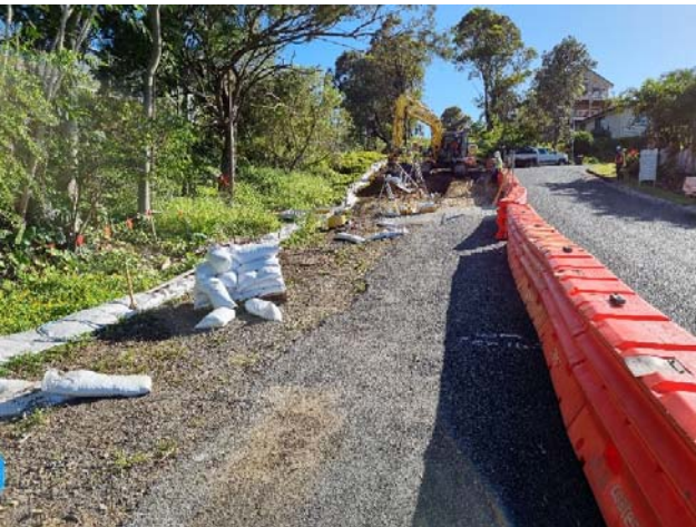
Image 3: Coachmans Close water main relocation (open trench excavation)
