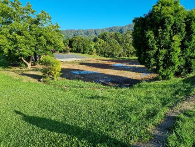
Image 1: Location of water main rupture environmental event 31/01/22 (Buchanans Rd)
