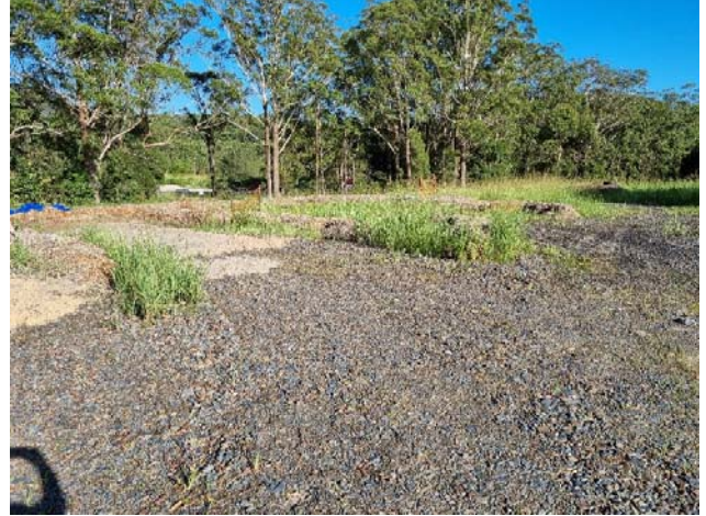
Image 2: Englands Rd Dewatering Area (mulch bund dewatering bays)
