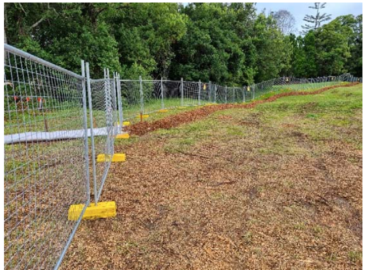
Image 4: Opal Blvd utility relocations (perimeter controls)
