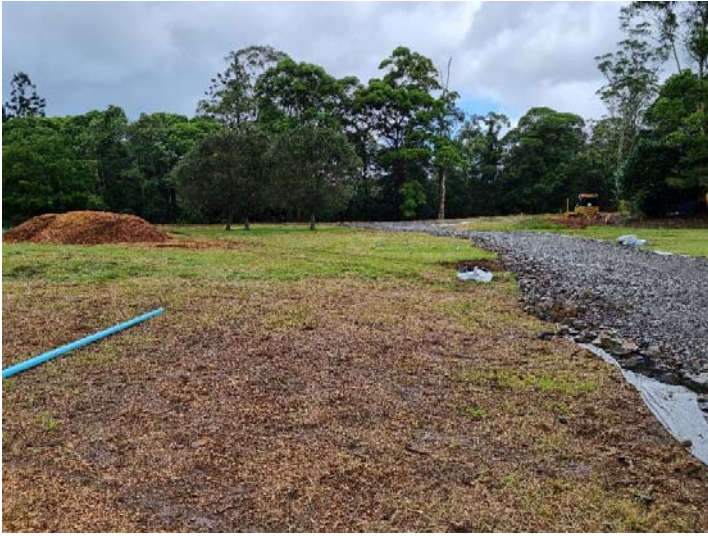
Image 5: Opal Blvd utility relocations (general view of work area)
