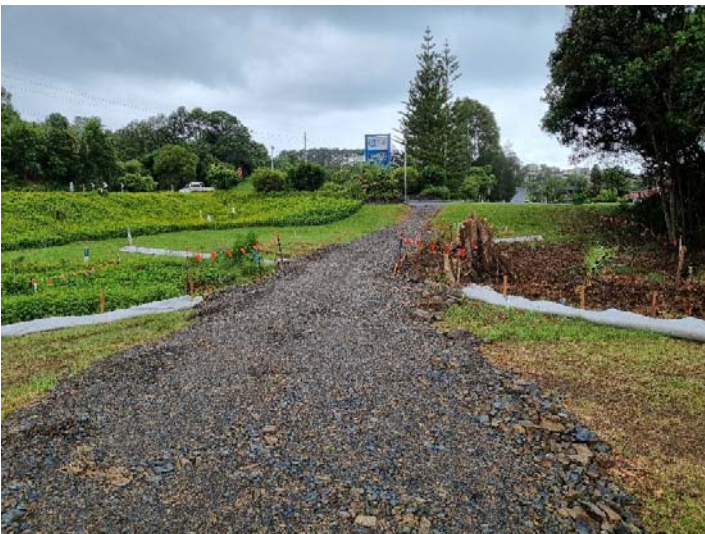
Image 3: Opal Blvd utility relocations (entrance to work area and waterway crossing)
