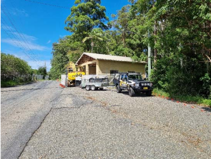
Image 1: Property demolition works (old RFS shed, Old Coast Rd)
