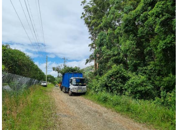
Image 2: Vegetation clearing works in preparation for utilities relocations (Old Coast Rd)
