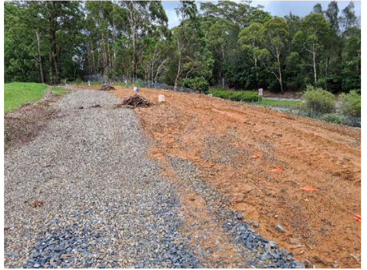
Image 6: Stadium Dr utility relocations – commencement of site clean-up
