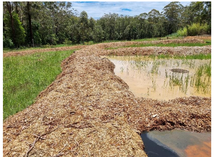
Image 4: Englands Rd Dewatering Area (dewatering bays formed using mulch bunds)
