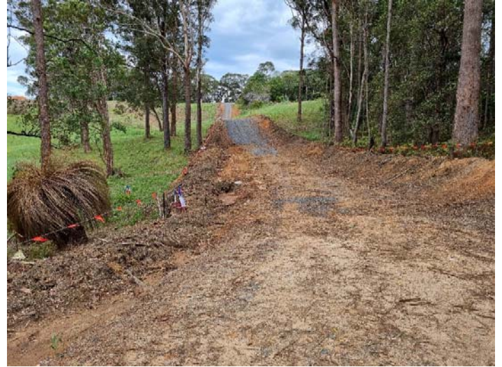
Image 2: Stadium Drive Utility Relocations
