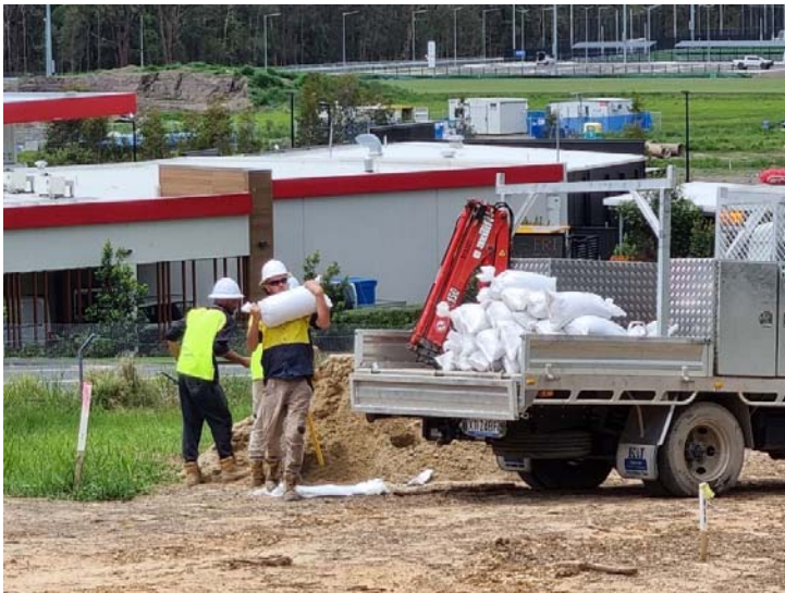
Image 3: Stadium Dr Utility Relocations – preparation for rain
