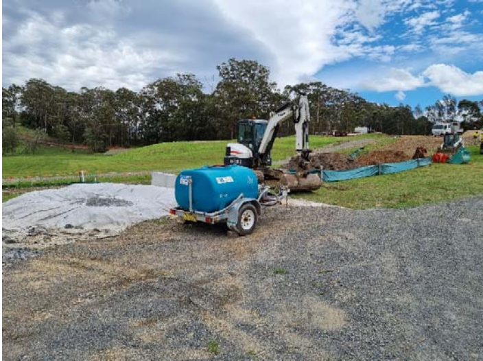
Image 1: Stadium Drive Utility Relocations
