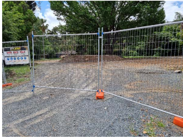
Image 6: Example house demolition site
