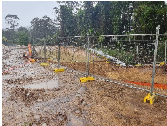
Image 6: North Boambee Road Utility Relocations
