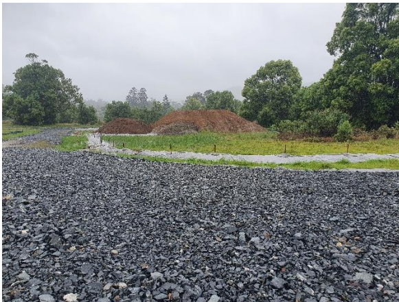
Image 5: North Boambee Road Utility Relocations
