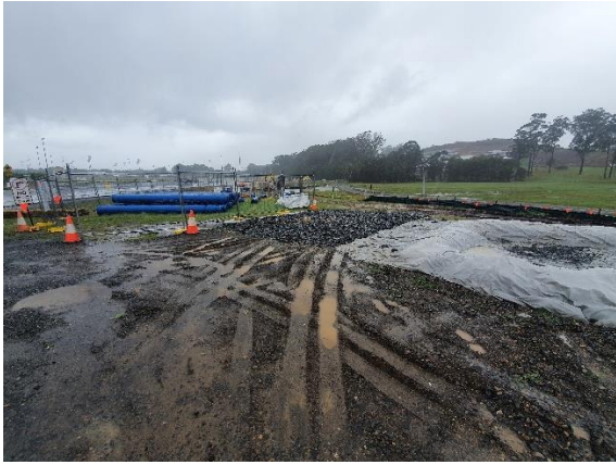
Image 1: Stadium Drive Utility Relocations
