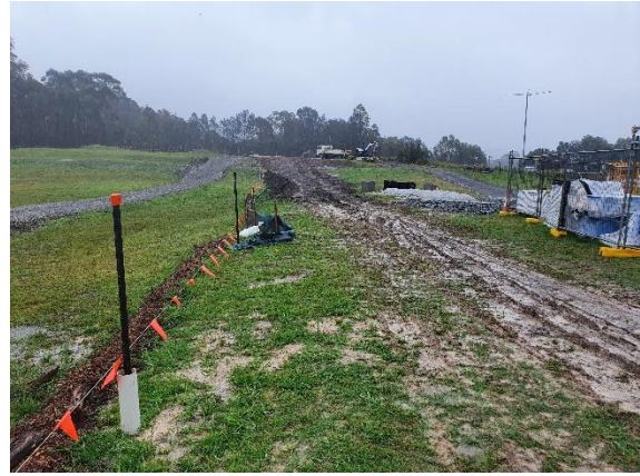
Image 2: Stadium Drive Utility Relocations
