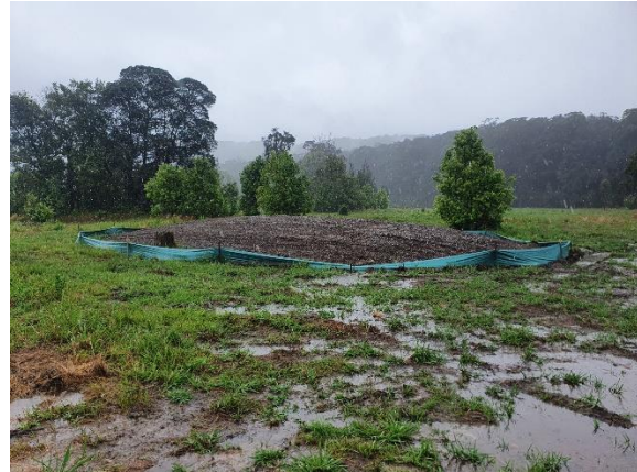
Image 4: North Boambee Road Utility Relocations
