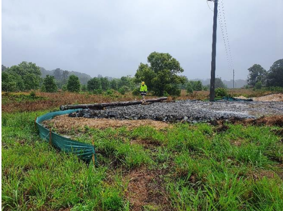
Image 3: North Boambee Road Utility Relocations
