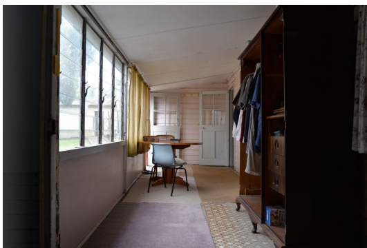
Figure 15. East facing view within the sunroom of the Former Coffs Heights Post Office. Note the modern building materials including metal frames glass louvre windows and plywood paneling on walls and ceiling
