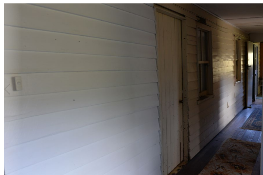
Figure 18. Northeast facing view within hallway showing original external weatherboard walling, timber panelled door and timber framed four panelled glass windows (now internal) of Former Coffs Heights Post Office
