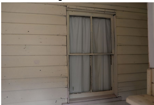
Figure 17. North facing view of original timber framed four panelled glass window (now internal) of Former Coffs Heights Post Office
