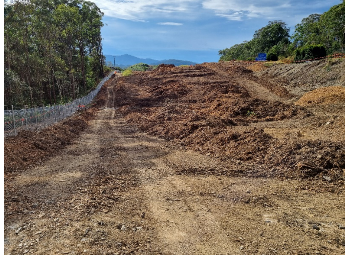
Image 2: South of Englands Rd (Ch10100 - 10800) – Vegetation clearing completed, mulch stockpiles
