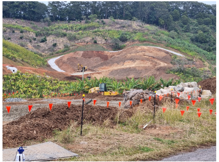
Image 6: Gatelys Rd tunnel portal north (Ch19300 - 19750) – Initial earthworks and clean water diversion drains
