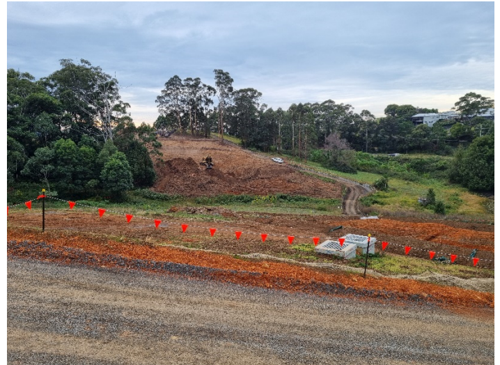
Image 8: Korora Hill Interchange (Ch20700 - 21300) – Mulching of cleared vegetation
