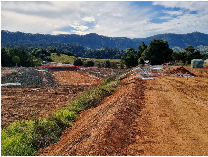
Image 5: Coramba Rd south (Ch14500) – Recently constructed sediment basin and vehicle washbay
