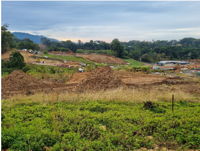
Image 7: Korora Hill Interchange (Ch20600 - 20900) – Vegetation clearing and ongoing utilities installation
