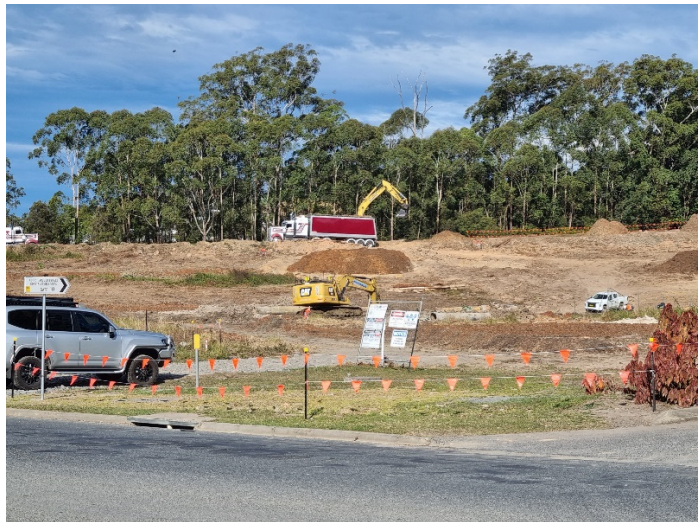
Image 3: Englands Rd Interchange (Ch10800) – Loading of mulch into trucks
