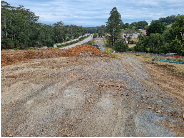
Image 1: Southern end of project (Ch9700 - 10100) – Vegetation clearing completed, mulch stockpiles
