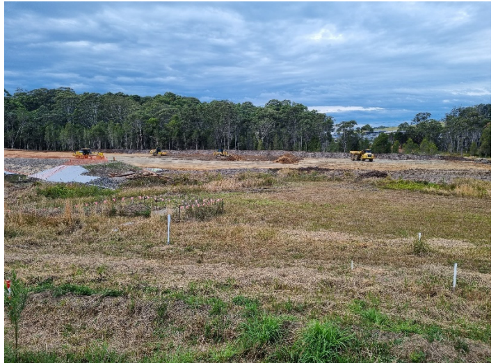
Image 4: North Boambee Rd, adjacent to compound (Ch12600 - 12800) – Earthworks
