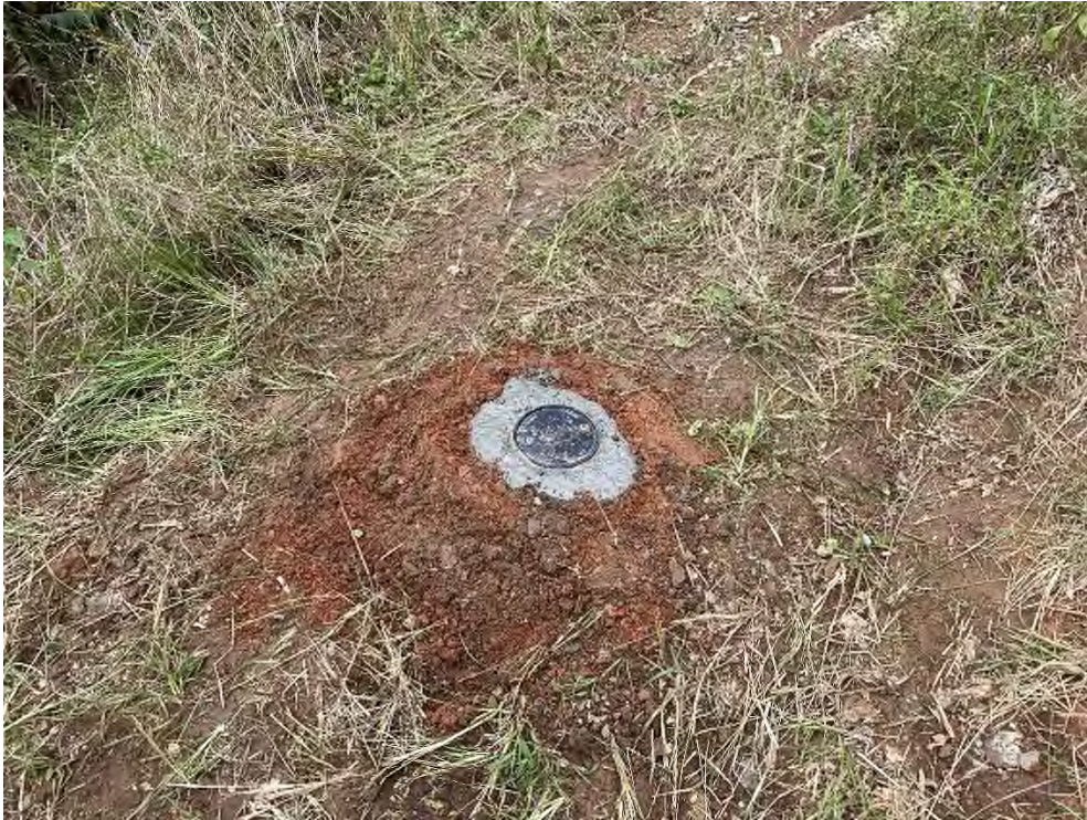
Photograph 5 , shows an example of a well repair for location BH2038, to the southeast of the Shephards lane tunnel.
