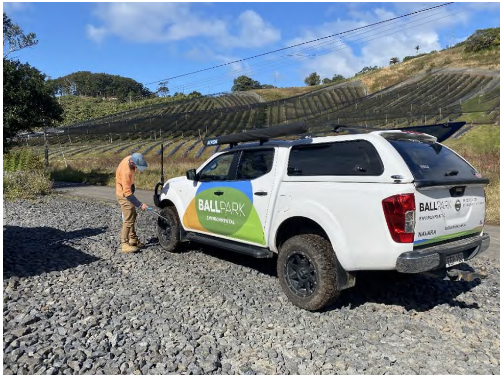
Photograph 6 , shows example of Panama disease decontamination undertaken of field vehicle using a Path X disinfectant spray. Location is the gravel wash down pad constructed to the north of Gatelys Road tunnel.
