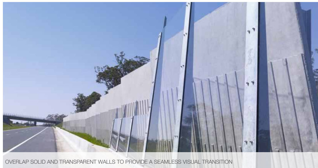
THE DESIGN SHOULD COMPRISE STEEL POSTS WITH TRANSPARENT PANELS.
