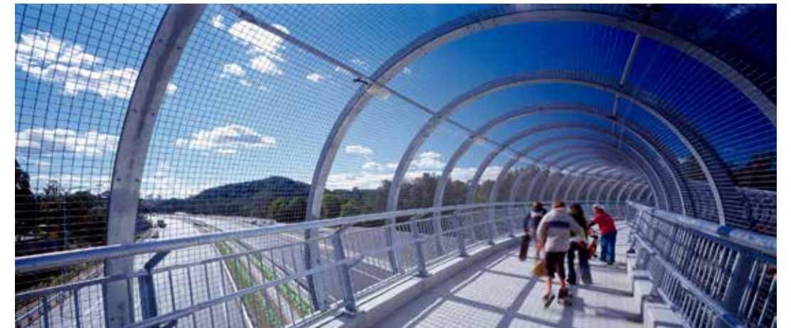
ENCLOSED SCREEN ON LLOYD PONTING SHARED PATH BRIDGE AT BILLINUDGEL RETAINS FEELING OF OPENNESS.
