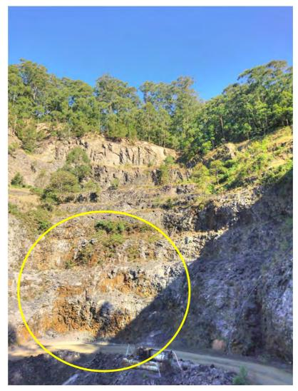
Photograph 9Groundwater seepage from shear zone in batter of TG Jungs<br/>Bennetts Road Quarry with dry batter faces on either side
