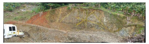
Photograph 6 Non planar/cross cutting shear zones (Wally Basarto's quarry) highlighted in yellow.
