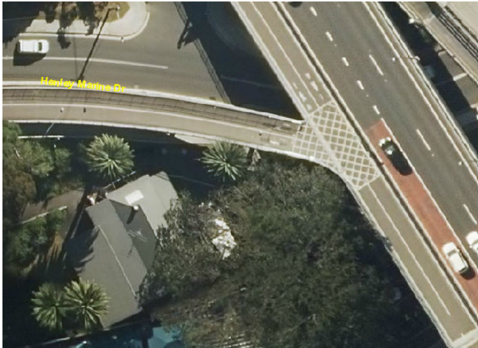
FIGURE 3 - HENLEY MARINE DRIVE AT VICTORIA ROAD, DRUMMOYNE - EXISTING SHARED/SEPARATED PATH TRANSITION
