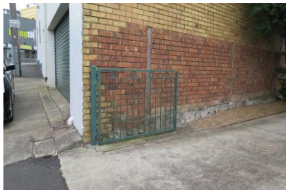
Figure 2-38 Looking north at the southwest corner of 224 Victoria Street The rear wall of the building has been constructed directly above bedrock (visible beneath the red brick section) (Source: GML 2016)
