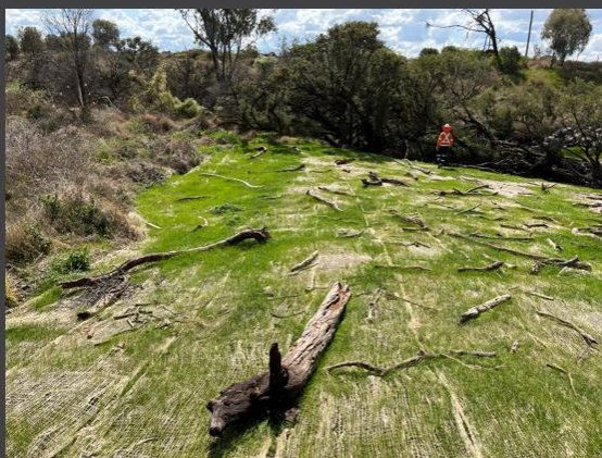
Croppa Creek – Woody debris disburshed throughout riparian zone as part of Creekside rehabilitation works – Note potential for augmentation of riparian zone function by planting trees and tall shrubs close to the creek line
