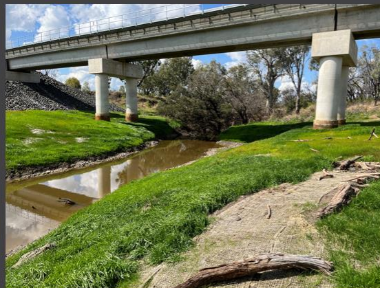
Croppa Creek – Woody debris disburshed throughout riparian zone as part of Creekside rehabilitation works – Note potential for augmentation of riparian zone function by planting trees and tall shrubs close to the creek line
