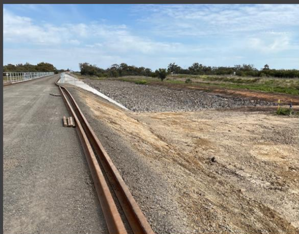
Final profile in Stage 2 – Awaiting Application of hydro mulch
