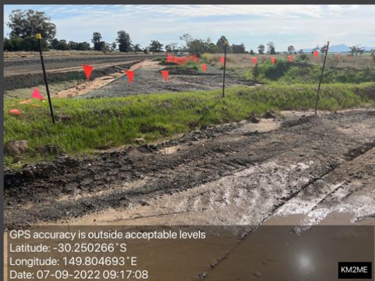
Gate 2b – Temporary soil stabilisation works
