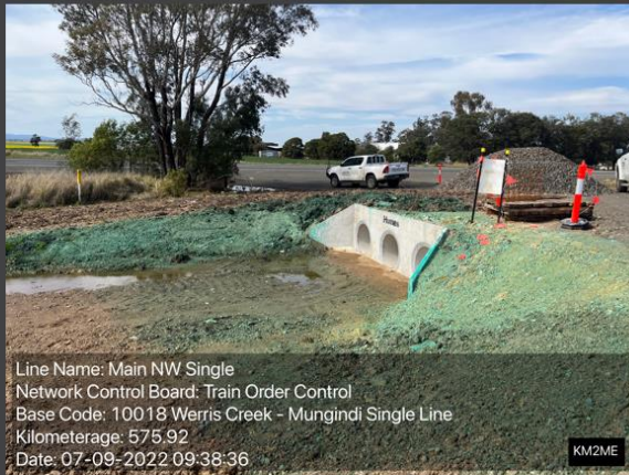
Soil binder application at Gate 1
