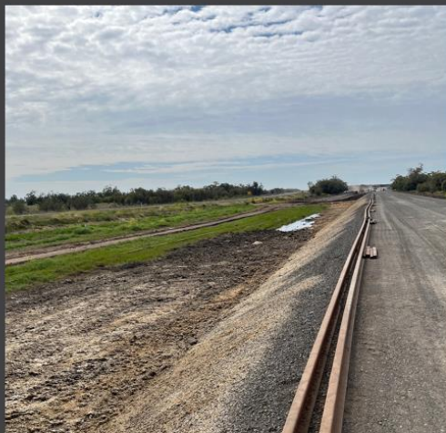
Final profile in Stage 2 – Awaiting Application of hydro mulch
