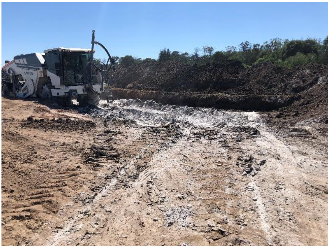
Plate 20 – Lime mixing along alignment
