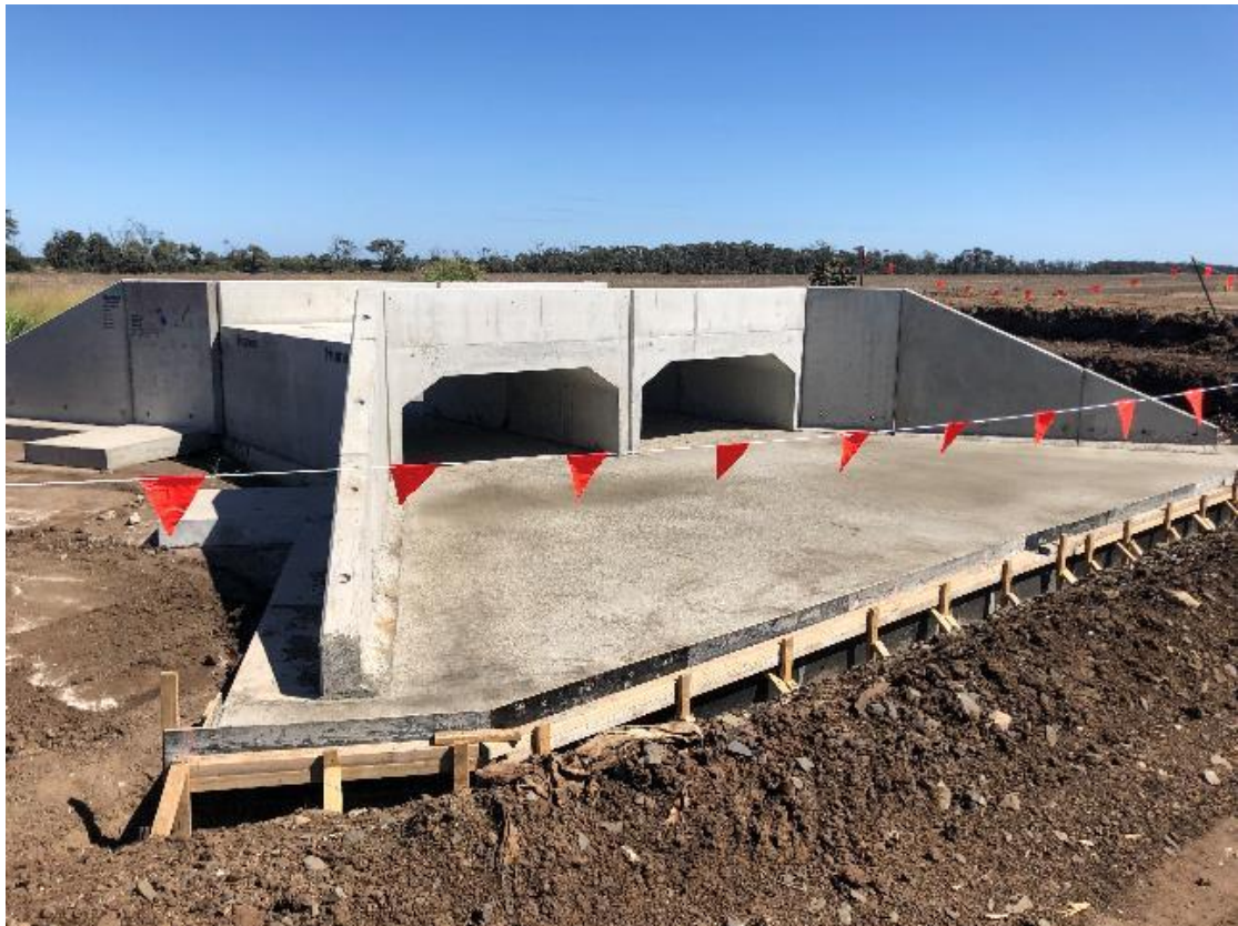
Plate 19 – Culverts installed along alignment – Chainage 736
