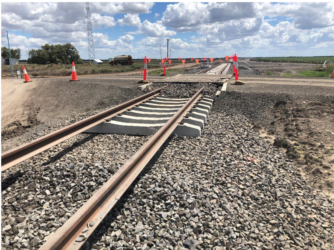
Plate 34 – Roydon Road Crossing and track installed
