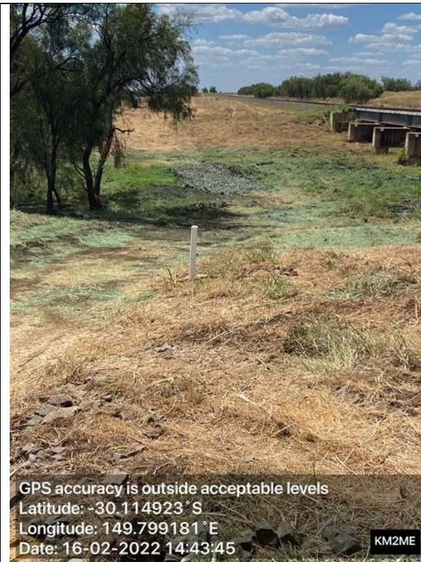
Soil binder applied to track leading down to creek
