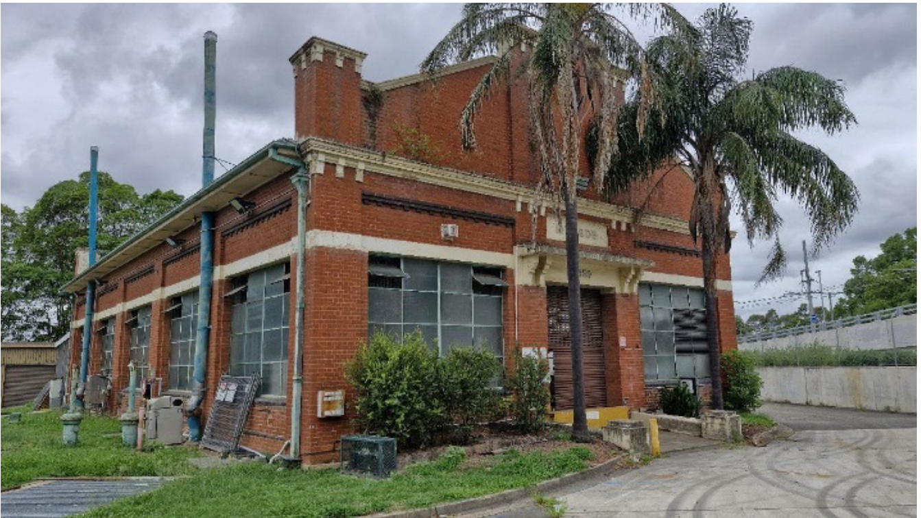
Plate 6.11 Sewage Pumping Station 067 structure. View south-east.
