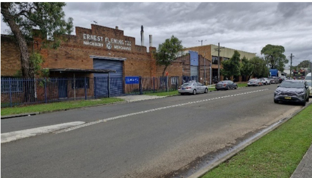
Plate 6.22 Ernest Fleming Pty Ltd Machinery Merchants on the north side of Derby Street. Pipeline alignment located under the south side of the road, opposite to the heritage structure. View, north-east.
