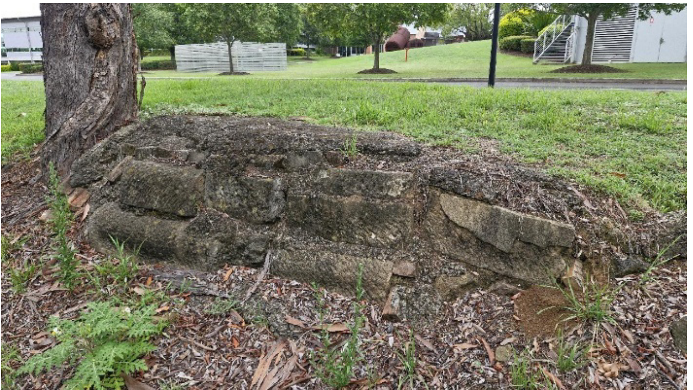
Plate 6.6 Sandstone and brick feature. View west.
