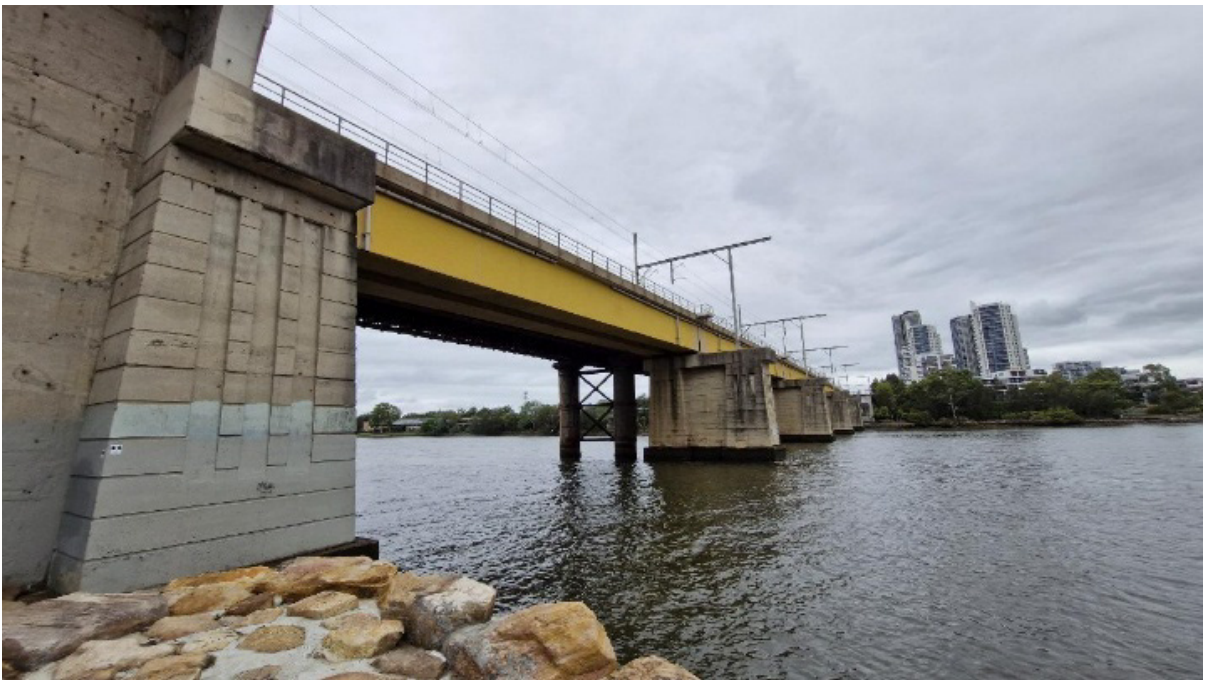
Plate 6.33 West side of Meadowbank rail bridge over Parramatta River. Indicative of river release pipeline alignment west of the bridge. View south-east.
