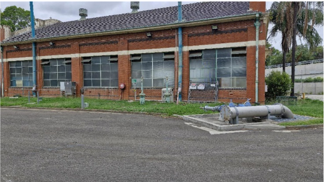
Plate 6.12 North side of Sewage Pumping Station 067 structure in background with pipeline alignment in the foreground. View south.
