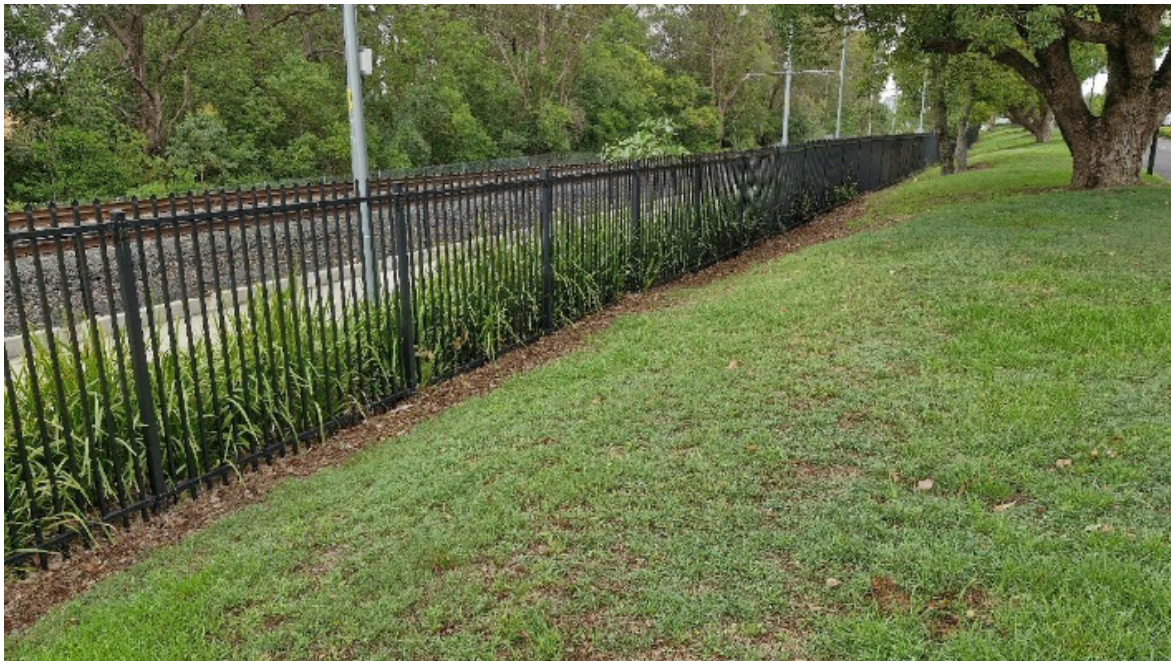
Plate 6.2 East curtilage of Rydalmere Hospital Precinct. View south-east.
