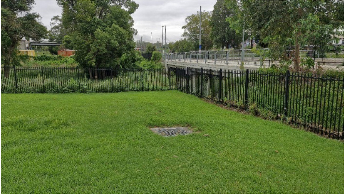
Plate 6.1 North-east corner of the Rydalmere Hospital Precinct curtilage. View north-east.
