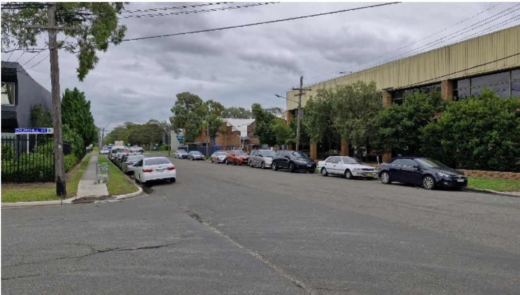
Plate 6.23 Location of pipeline alignment under the south side of road with the Earnest Fleming Pty Ltd Machinery Merchants structure on the north side of the road. View, north-west.
