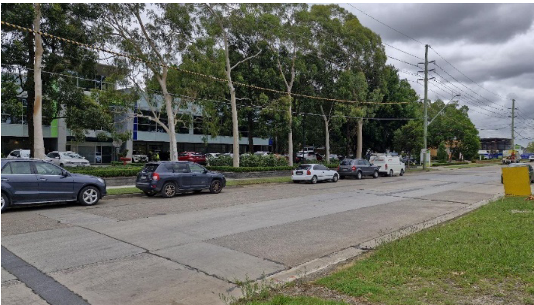
Plate 6.20 North curtilage of Capral Aluminium at Unwin Street. View south-west from WRRF.
