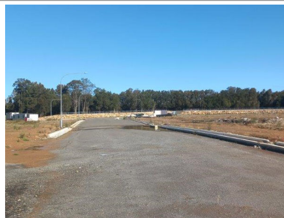
Photo 3 View south from the WRRF site towards 'Southern Buried Waste Area'.
