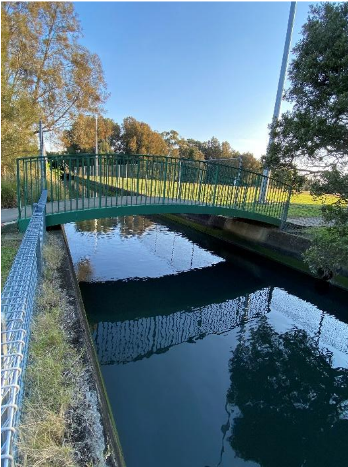
Figure 7-2: Existing footbridge crossing of Smalls Creek
