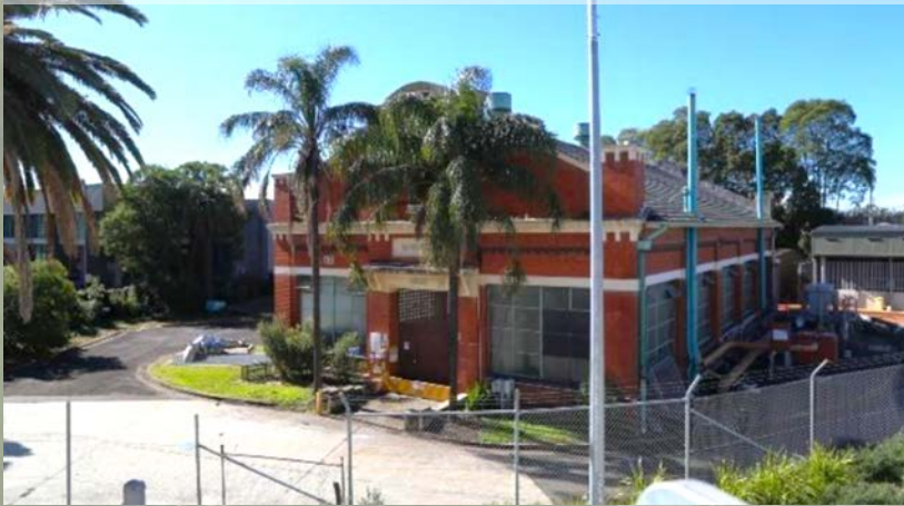
Overview of pumping station viewed from pedestrian walkway to south of site, looking north-east
