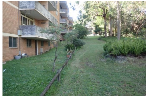
Plate 2. View to southeast at boundary of Memorial Park. Study area alignments runs upslope to Meadow Crescent, between Memorial Park (right) and a block of units, No.12 Meadow Crescent (left).
